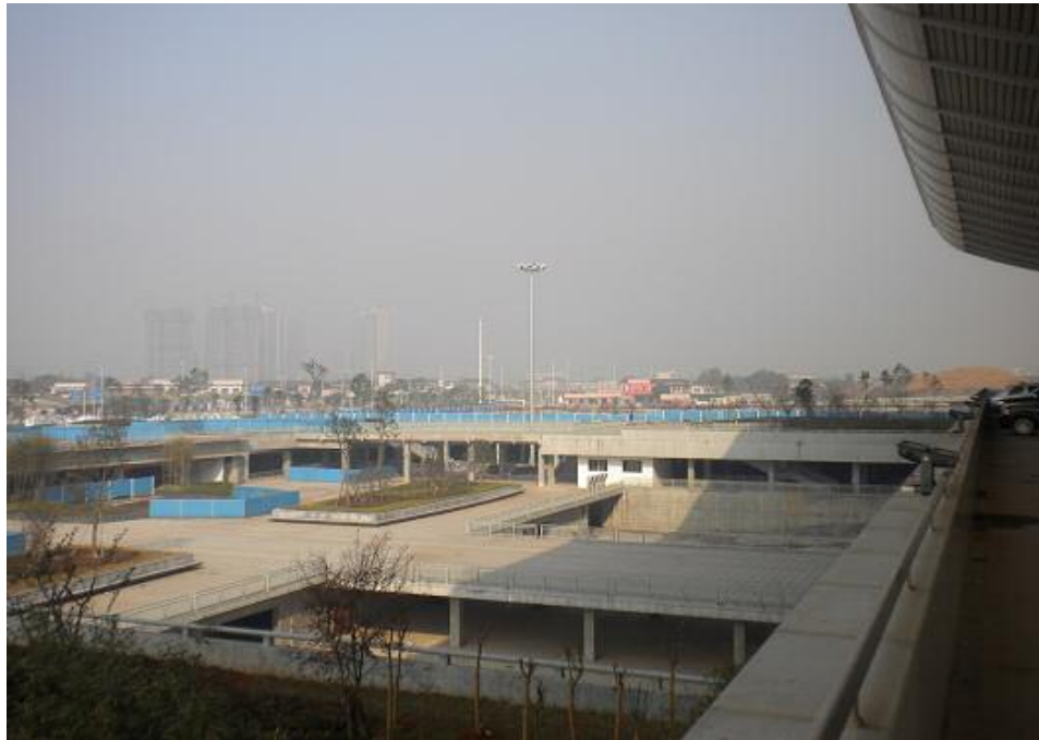
Figure 2-7 Underground area has been Constructed
