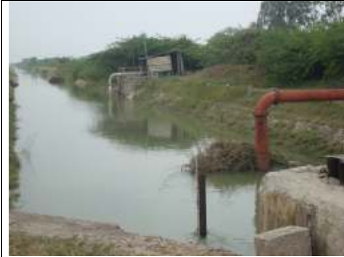
Intake of Left Bank canal ( Tungabhatra river)
