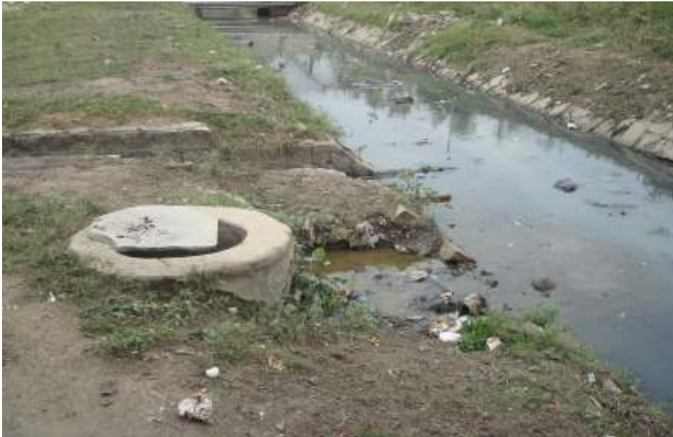
Figure 1: Sewage connecting to the nearby nallah behind IOC colony
