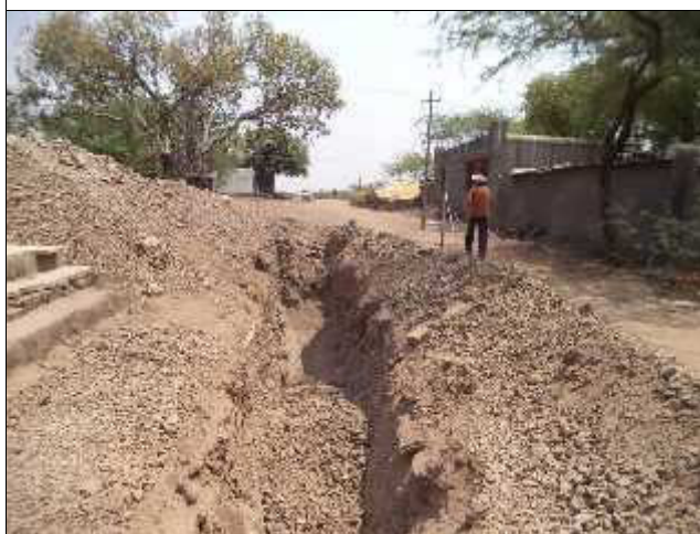
Trenching site without board, barricade and fencing
