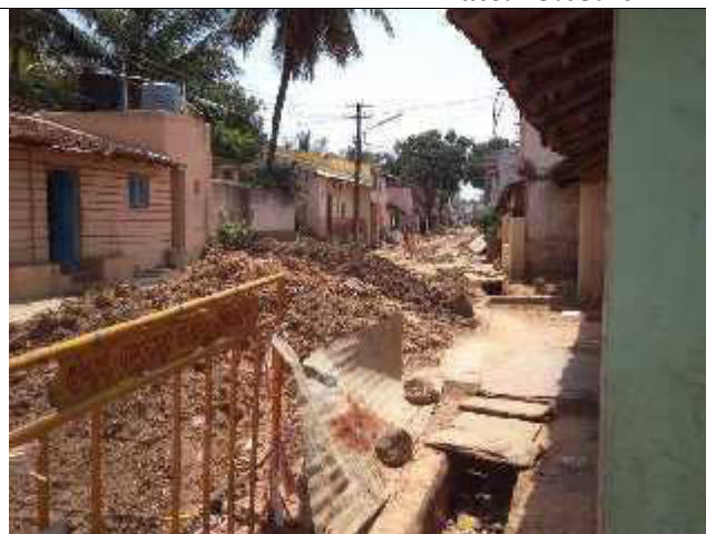
Side barricading provided partially
