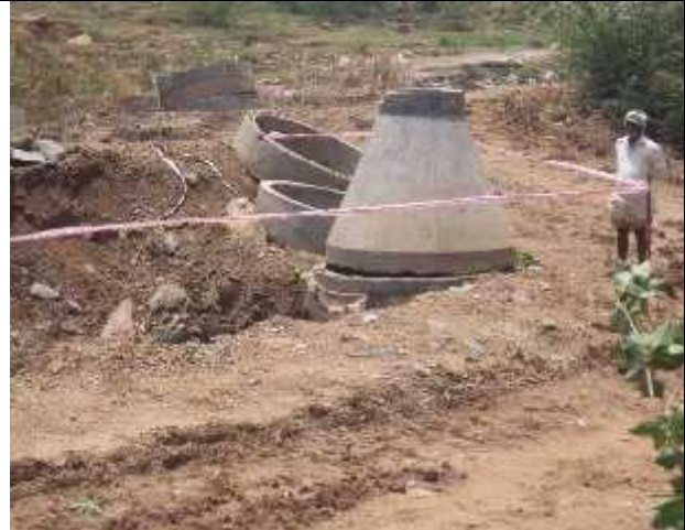
Caution tape provided at the excavation site
