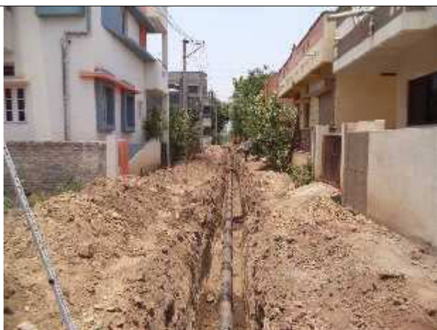
Trenching in residential area. No side protection
