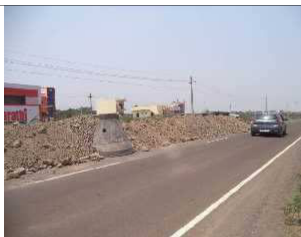
No caution board / tape, barricading
