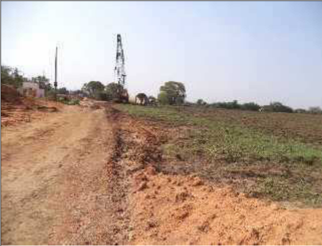
Excavated soil eroded into Agriculture land
