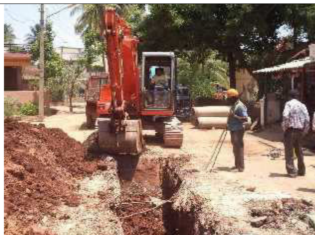
Side protection, barricade or tape not provided
