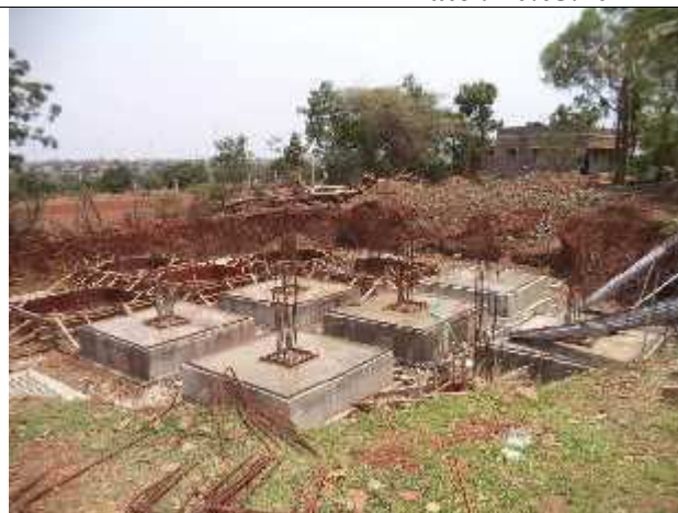
Excavation site without barricade or warning board.
