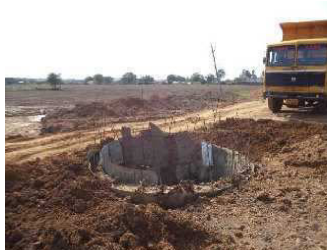
No Caution board or tape provided at trenching site
