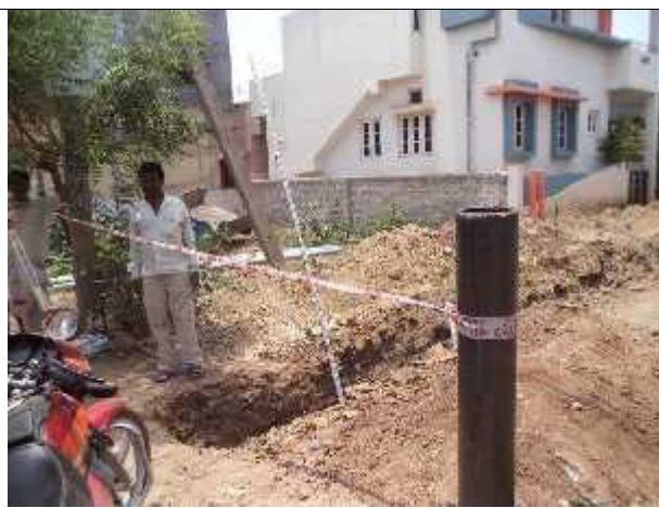
Caution tape provided partially at one end only
