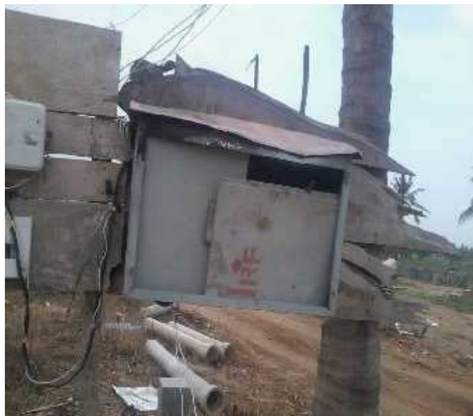
Exposed Panel board - unsafe practice
