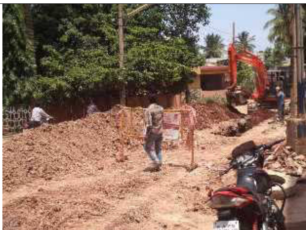
Caution board and barricade at the trenching site
