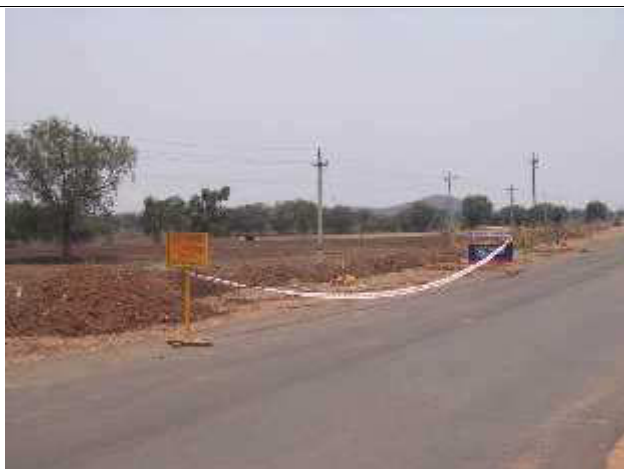
Barricade, Caution tape provided along the trench
