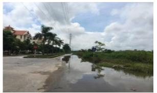
Flooded situation when the culvert is lower than road surface and it not frequently dredged
