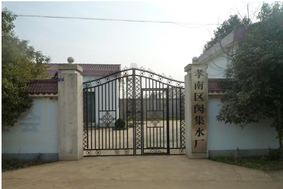
Figure 1.5-1 Current situation of Minji water plant
