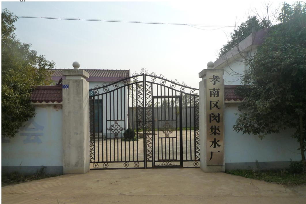
Figure 4 Minji Water Treatment Plant
