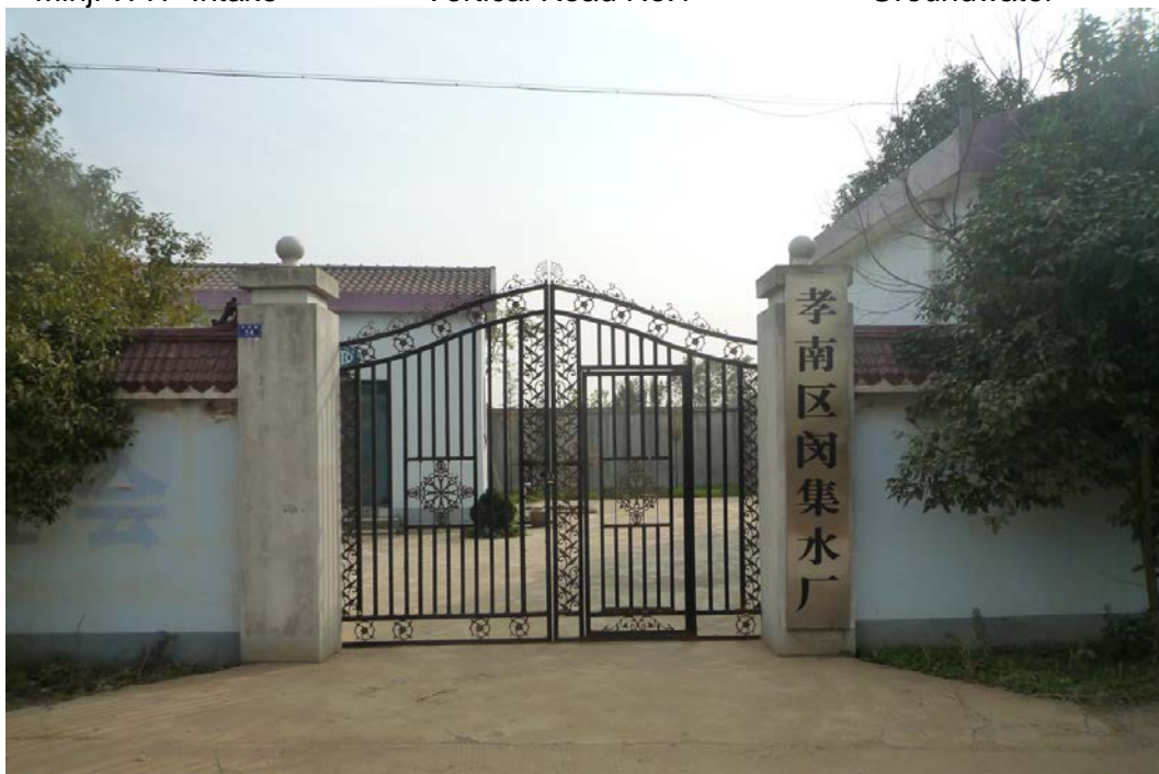
Figure 4 Minji Water Treatment Plant
