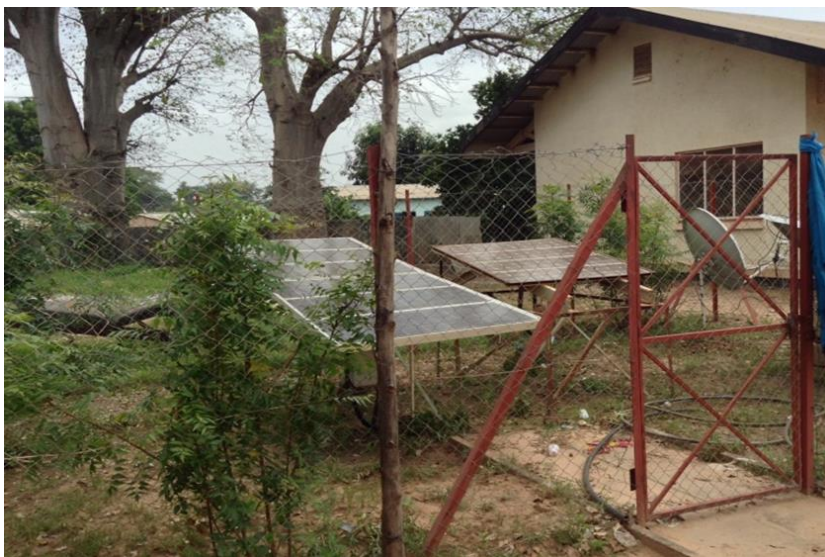
Solar panels within Kuntaur Health Centre
