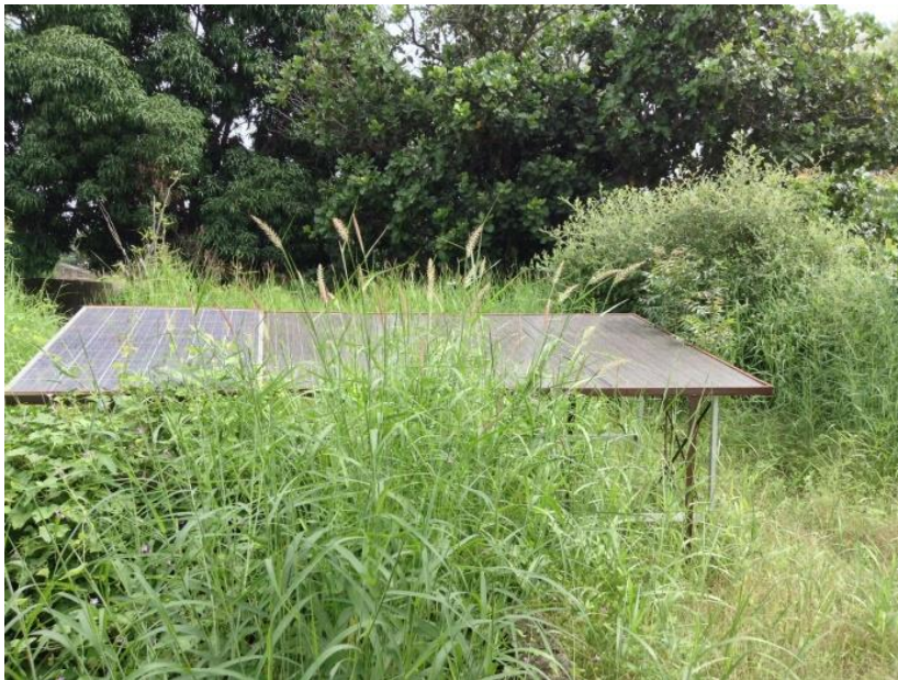
Non-operational solar panels at Farafenni Upper Basic School
