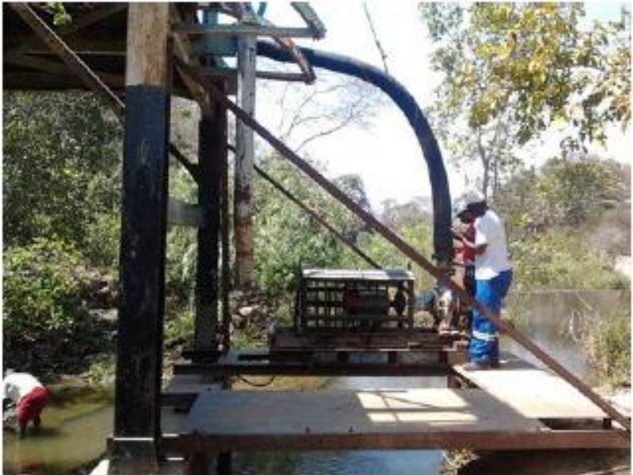
Figure 3:Raw water abstraction point
