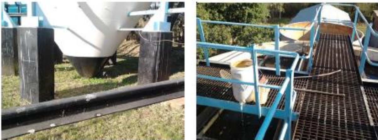
Figure 4: Water treatment unit
