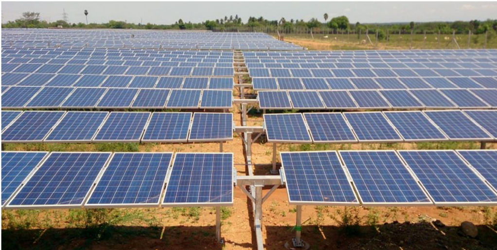
Figure 29: Single axis tracker system
