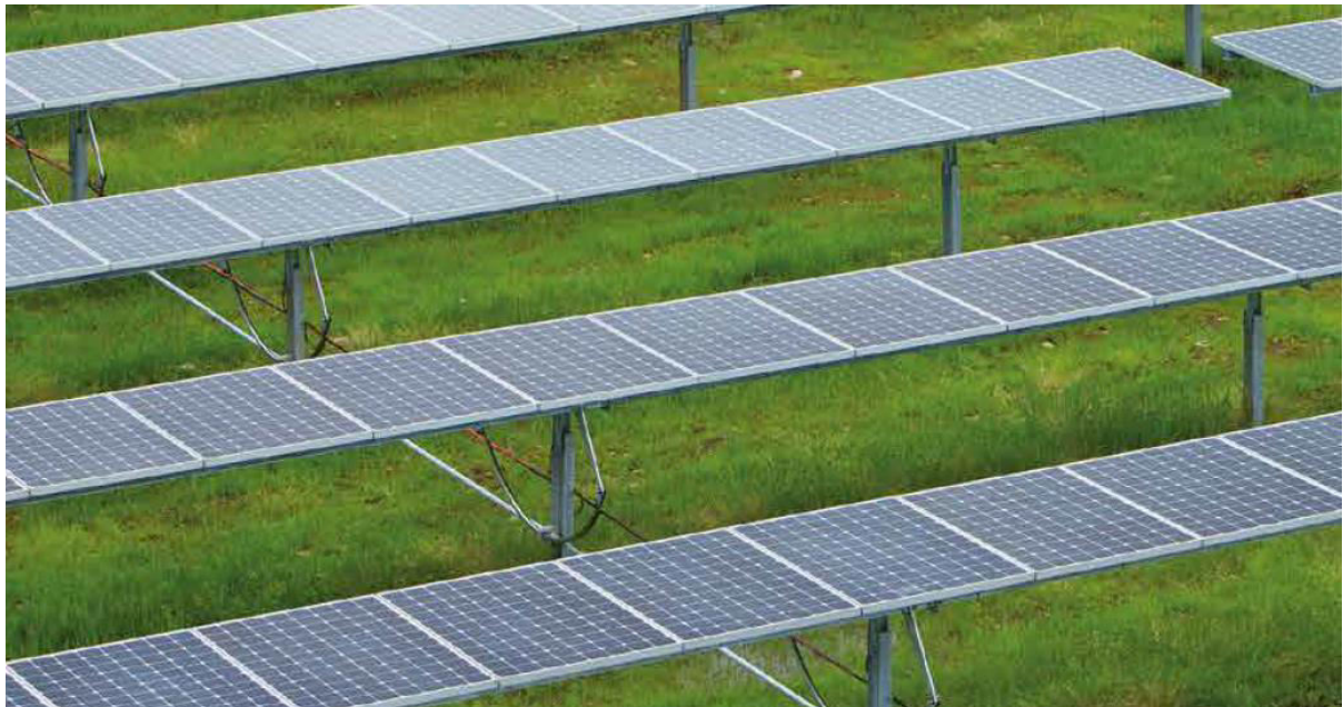
Figure 5 Mounted 1-axis tracker PV (example)
