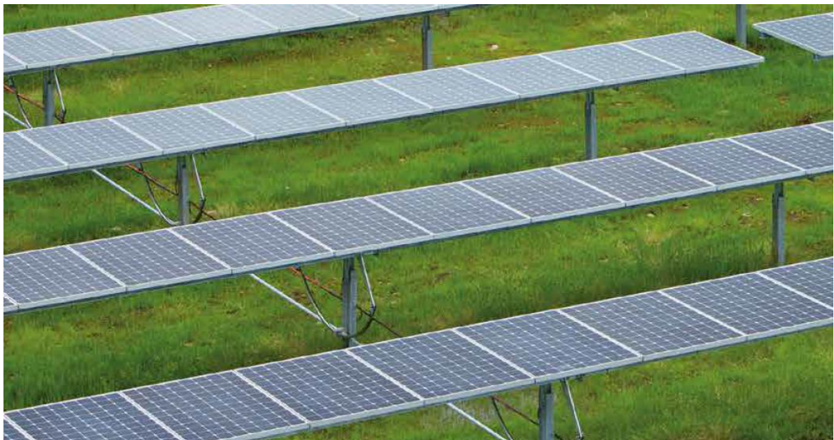
Figure 5 Mounted 1-axis tracker PV (example)
