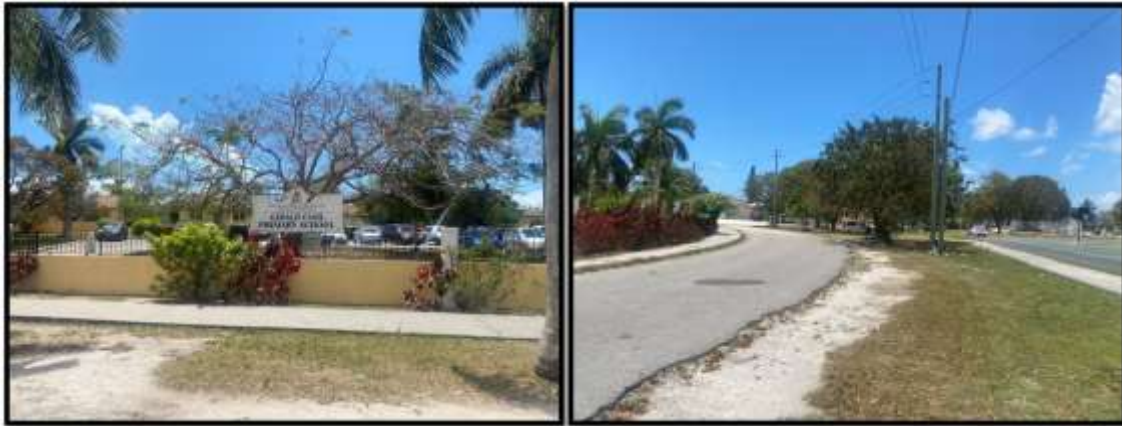
Figure 126. (a) Gerald Cash Primary School, adjacent to Lift Station on Flamingo Gardens Park; (b) Bangladesh Crescent Road. Source: PlanEHS, 2024.
