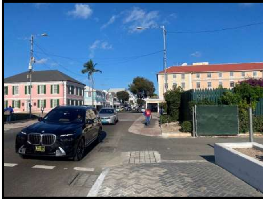
Figure 136. Bay Street with overhead lighting and sewer system and view of Rawson Square Lift Station (green fenced). Source: PlanEHS, 2024.
