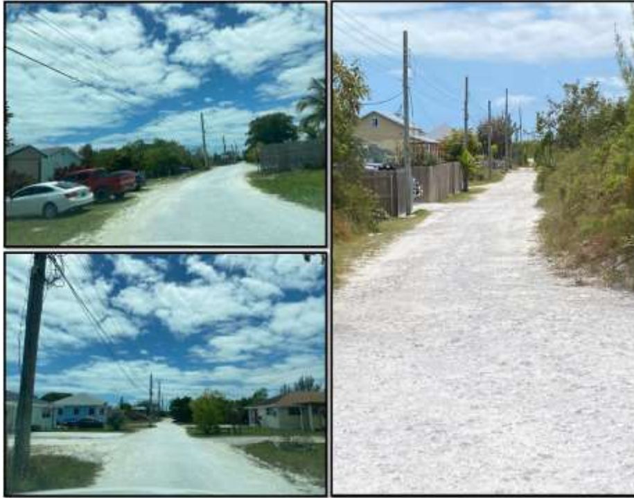
Figure 110. Overhead electricity poles in Sweetings Tract. Source: PlanEHS, 2024.
