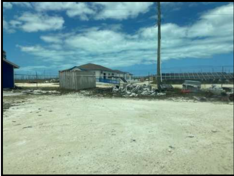
Figure 163. Pumping Station, Storage Building, Generator Building and Solar Plant. Source: PlanEHS, 2024.
