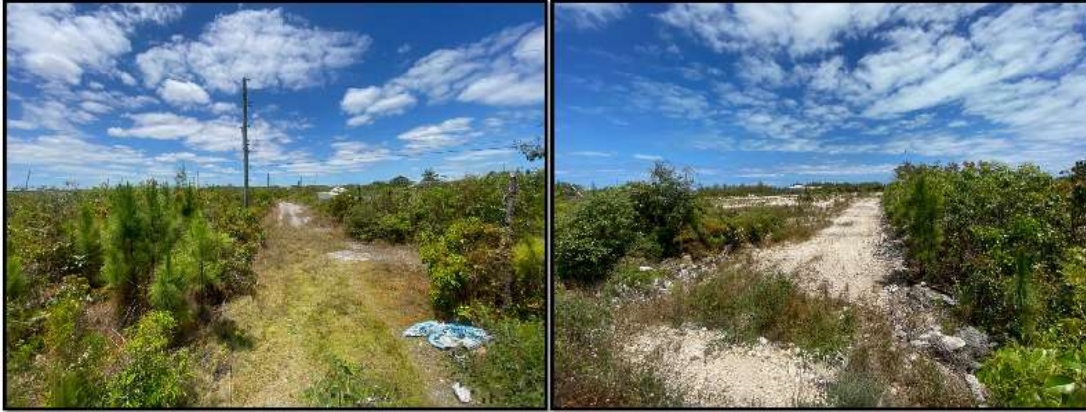
Figure 114. Uncleared and unpaved roads. Source: PlanEHS, 2024.
