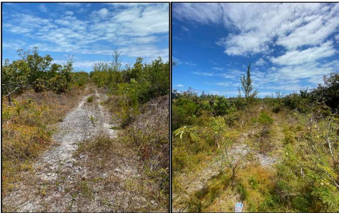
Figure 115. Uncleared and unpaved roads. Source: PlanEHS, 2024.
