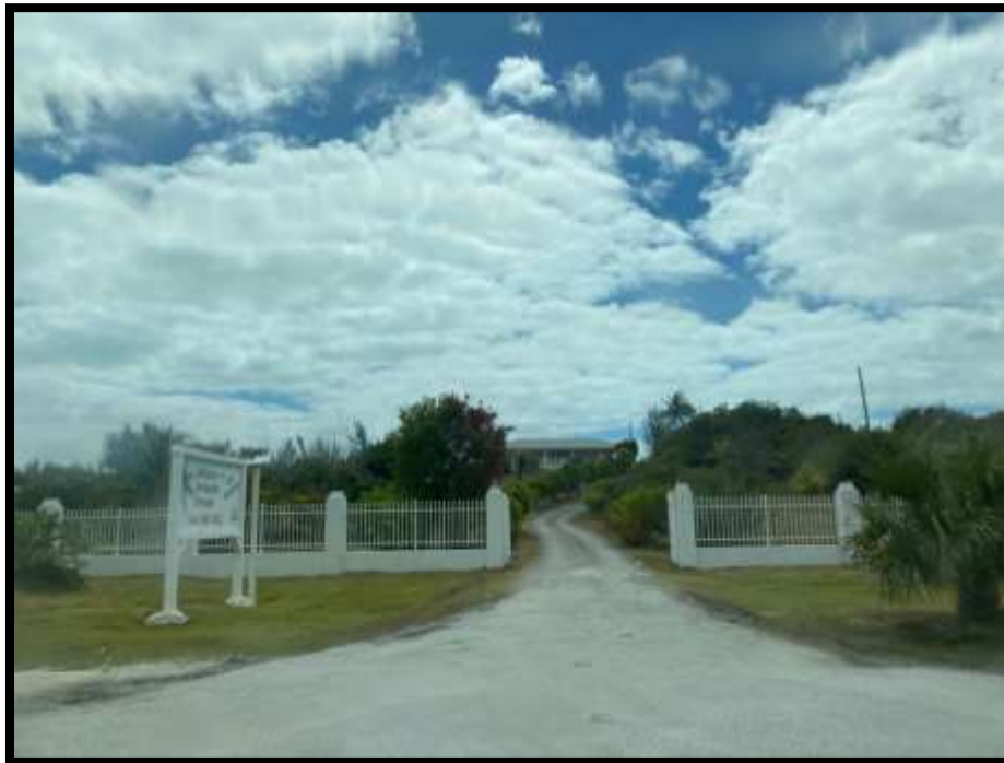
Figure 97. Abaco Hillside Hotel. Source: PlanEHS, 2024.
