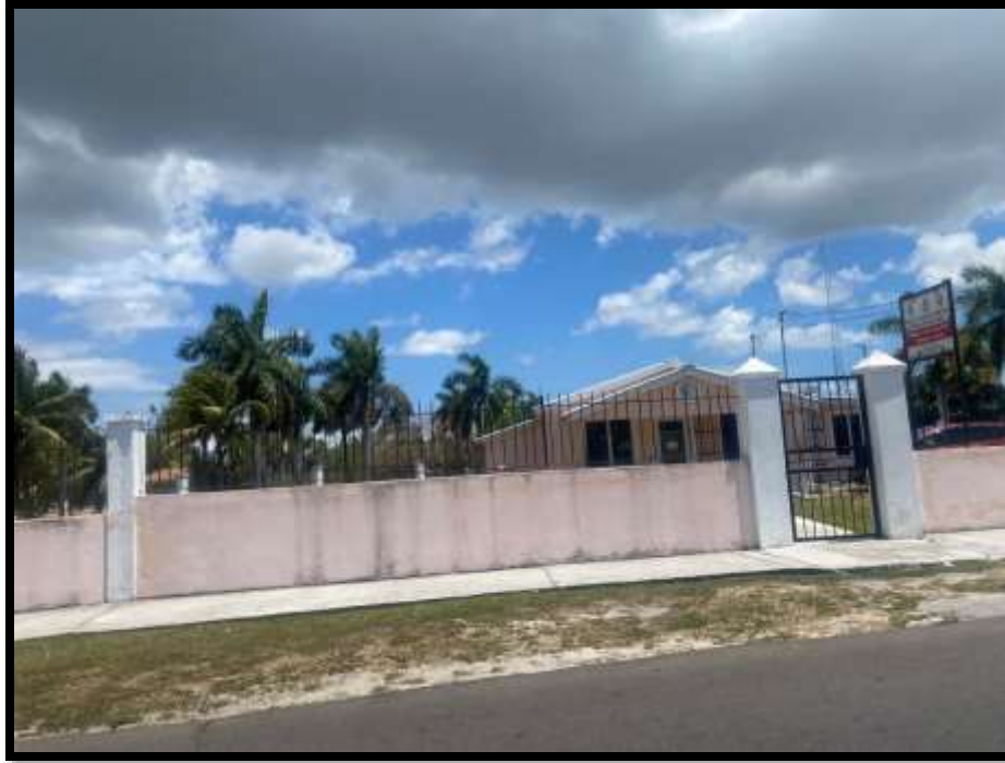
Figure 125. Ministry of Social Services & Urban Development 330ft from lift station. Source: PlanEHS, 2024.
