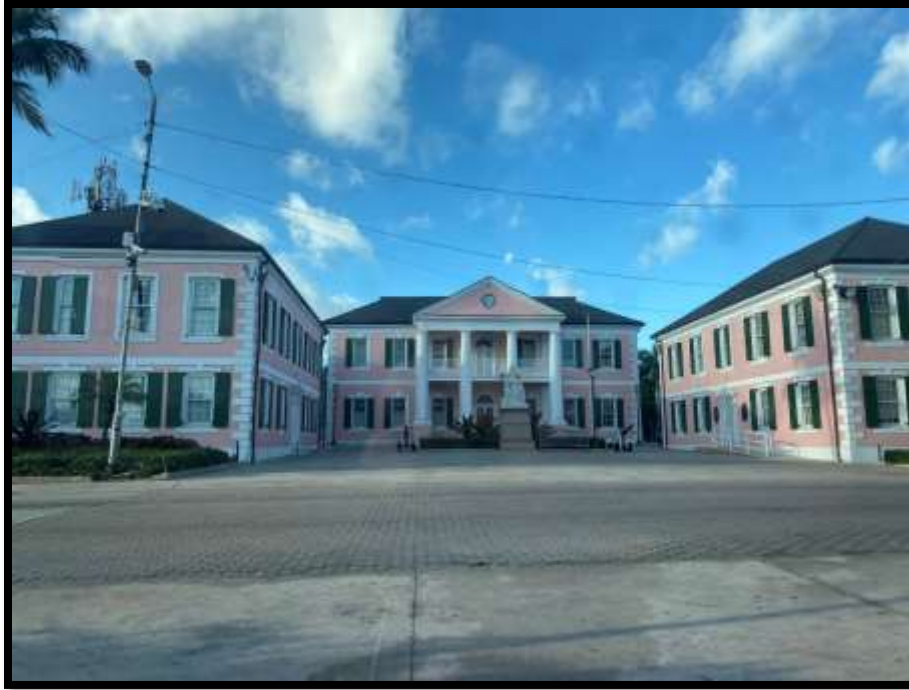
Figure 137. Parliament Square in front of Rawson Square Lift Station. Source: PlanEHS, 2024.
