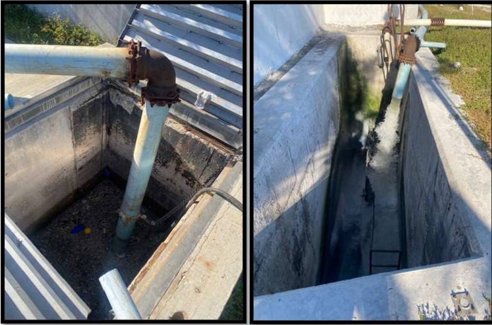
Figure 34. (a) 1 o well chamber and PVC bypass; (b) 2 o well chamber and PVC bypass. Source: PlanEHS 2024.
