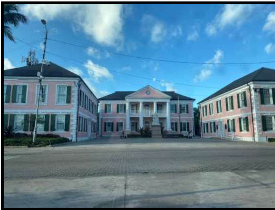
Figure 74. Parliament Square, Historical Buildings located in front of a proposed project site (Rawson Square Lift Station). Source: PlanEHS, 2024.
