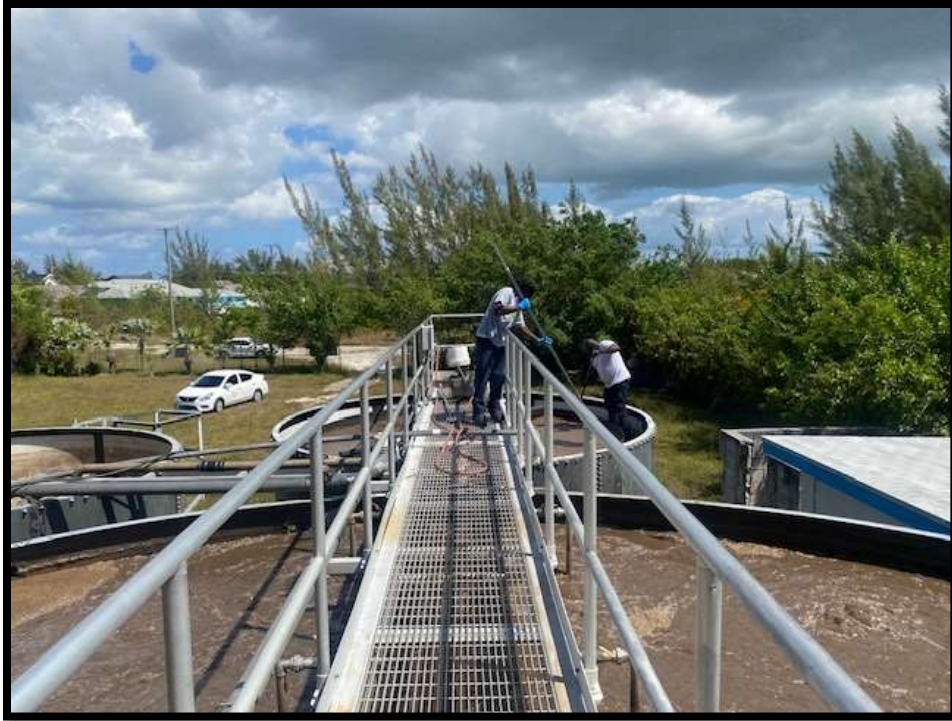
Figure 172. View of Aeration, Clarifier and Digestion Tanks. Source: PlanEHS, 2024.
