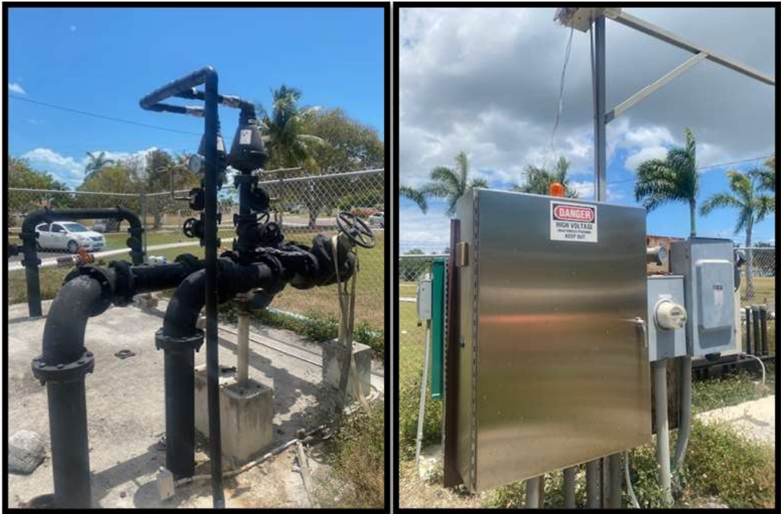
Figure 18. (a) Overground valves; (b) Pump Control Panel. Source: PlanEHS, 2024.
