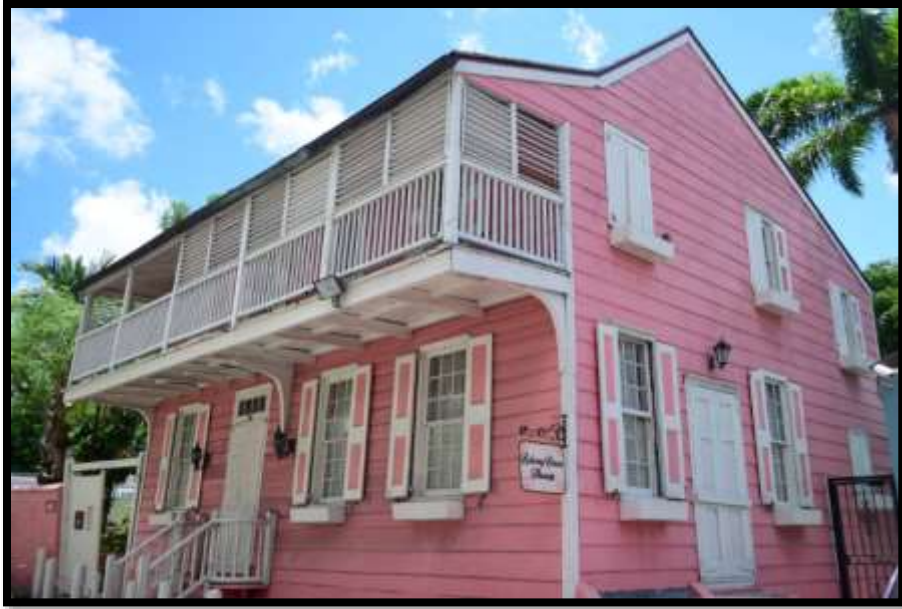
Figure 73 – Balcony House near a proposed project site (Rawson Square). Source: AMMC website
