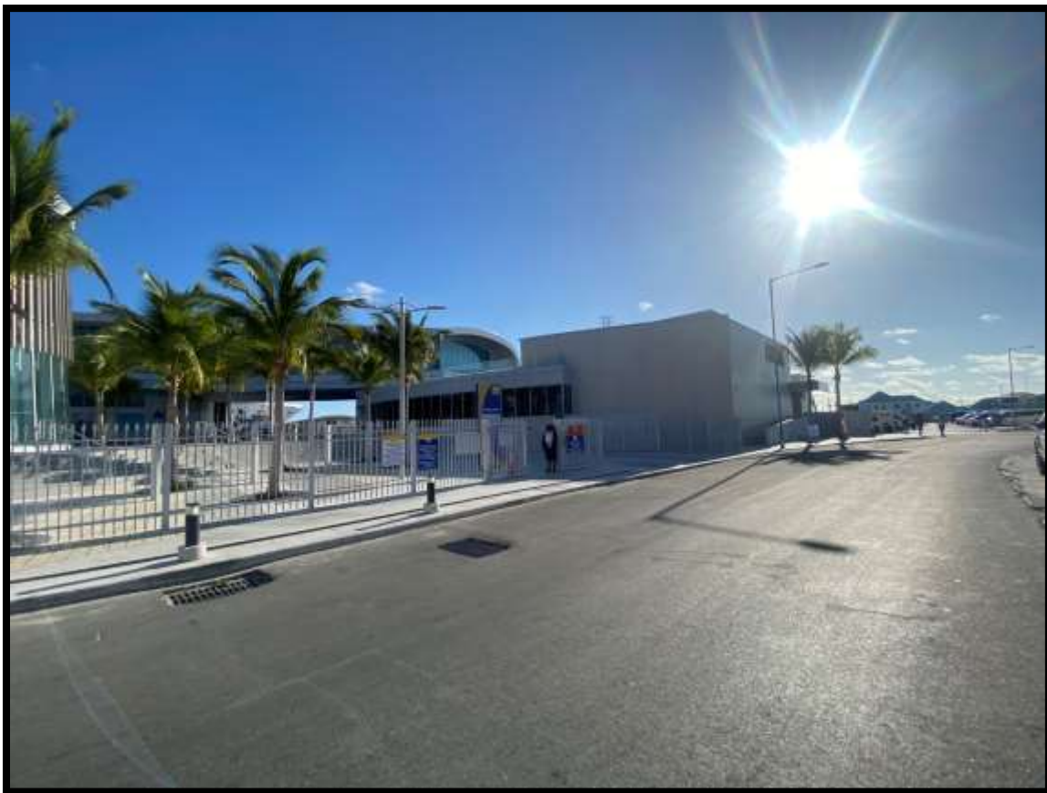
Figure 129. Bahamas Cruise Terminal, 130 ft from Rawson Square Lift Station. PlanEHS, 2024.
