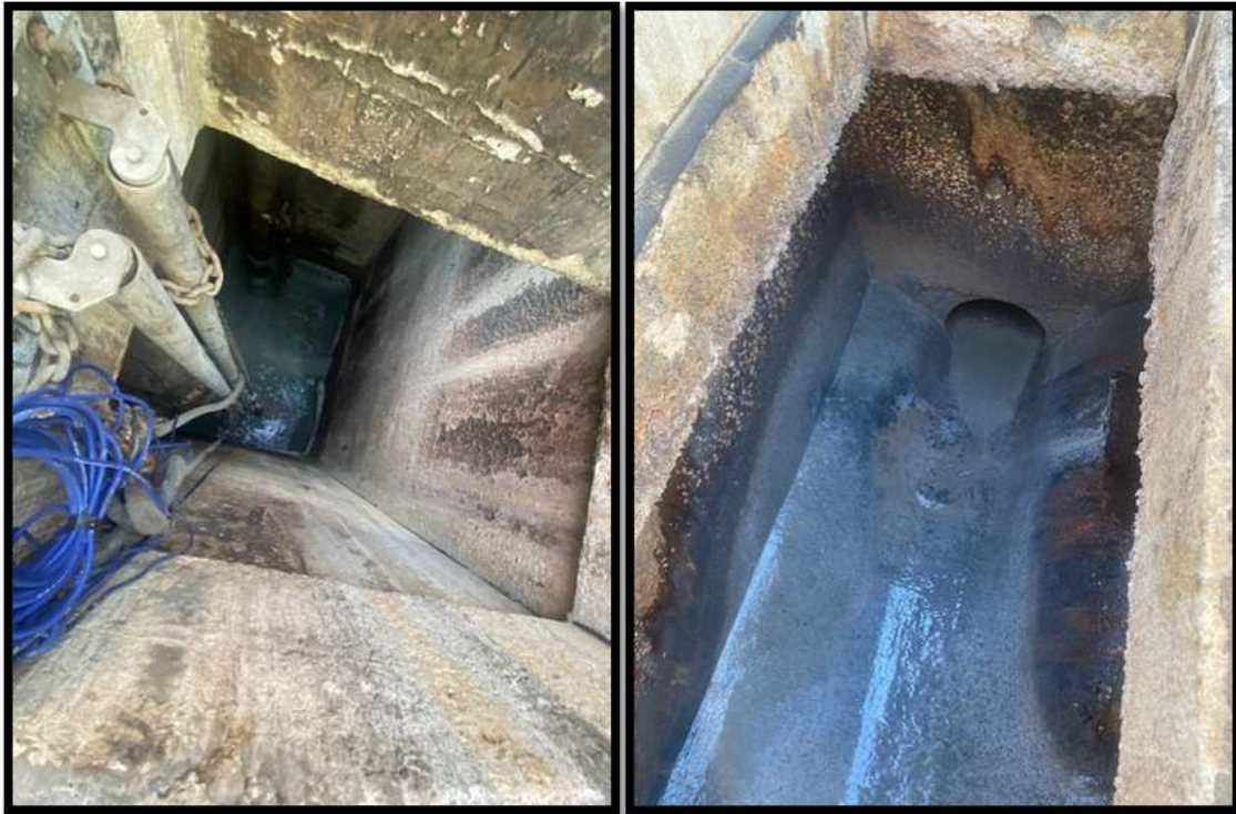
Figure 28. Well chamber and secondary chamber. Source: PlanEHS, 2024.
