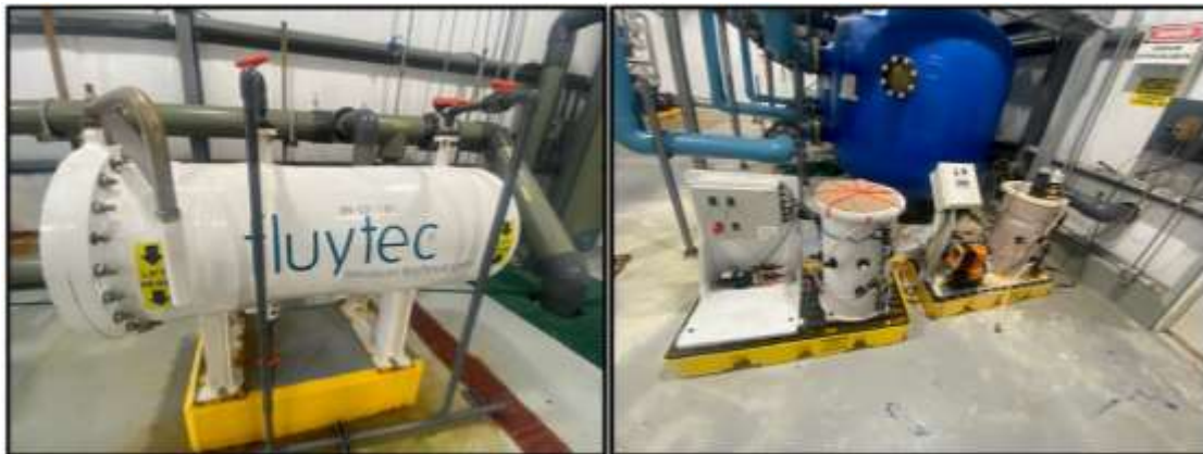
Figure 147. Potabilization Process: (a) Filtration prior to RO membranes; (b) Chlorination after RO process. Source: PlanEHS, 2024.
