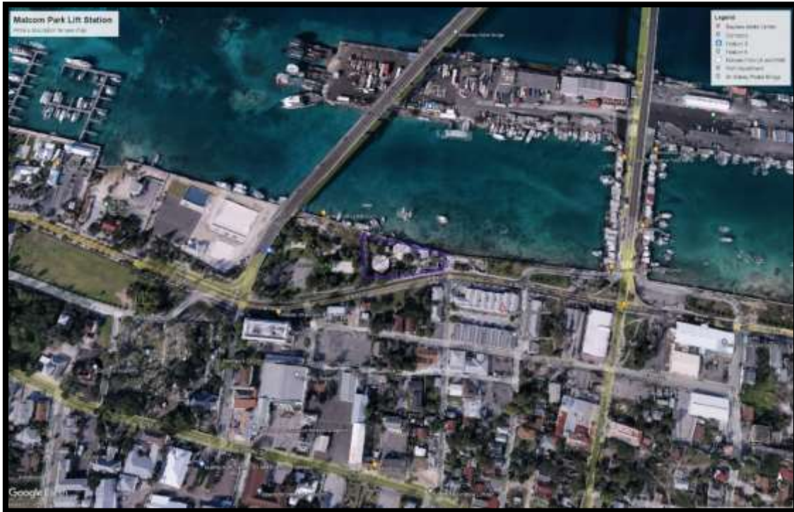
Figure 29. Malcom Park Lift Station (and well). Source: PlanEHS, 2024.
