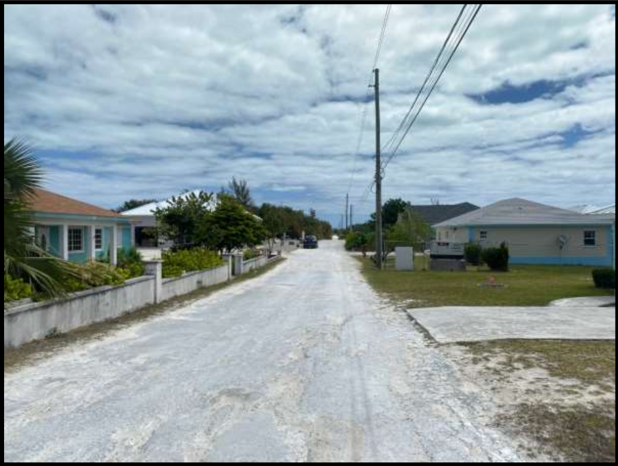
Figure 101. Residential houses and deterioration on paved roads.
