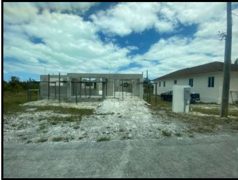
Figure 90. Development of the neighborhood, houses in construction. Source: PlanEHS, 2024.
