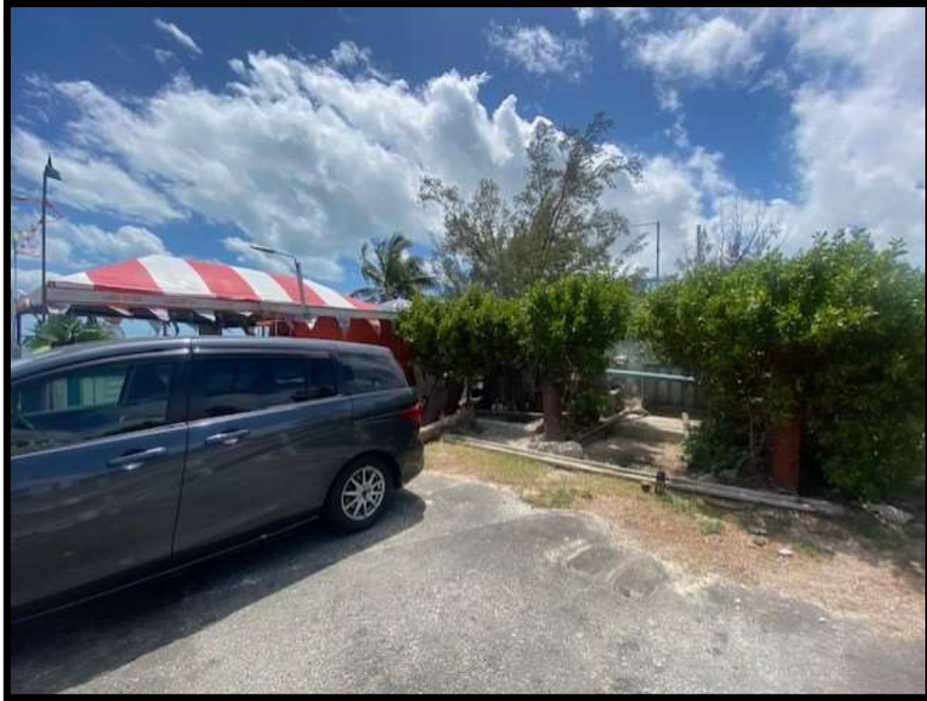
Figure 36. Location of Montague Lift Station, adjacent to local vendor. Source: PlanEHS, 2024.
