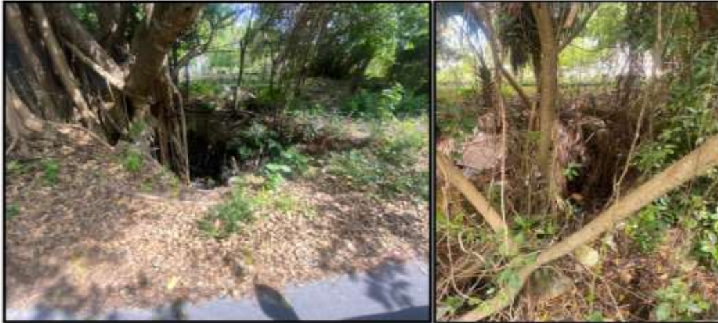
Figure 150. Sinkholes around RO Plant. Source: PlanEHS, 2024.
