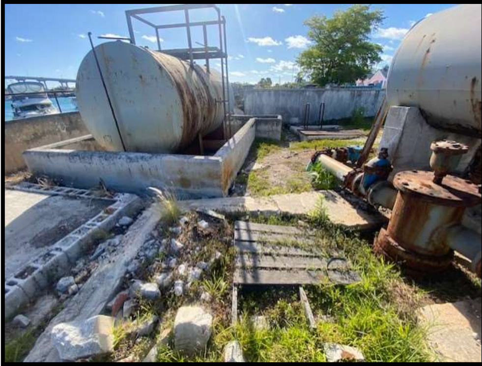
Figure 34. Injection well (right) and unused fuel tank (left) and screening tank (right). Source: PlanEHS, 2024.
