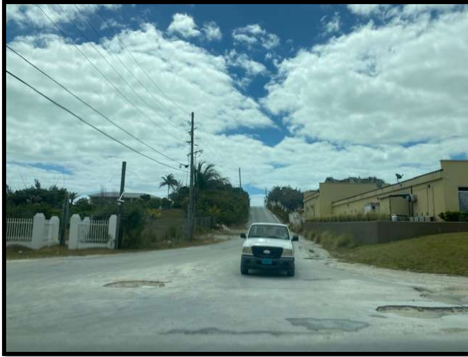
Figure 88. Entrance to Sweetings Tract, Great Abaco Highway and John Sweetings Drive. Source: PlanEHS, 2024.
