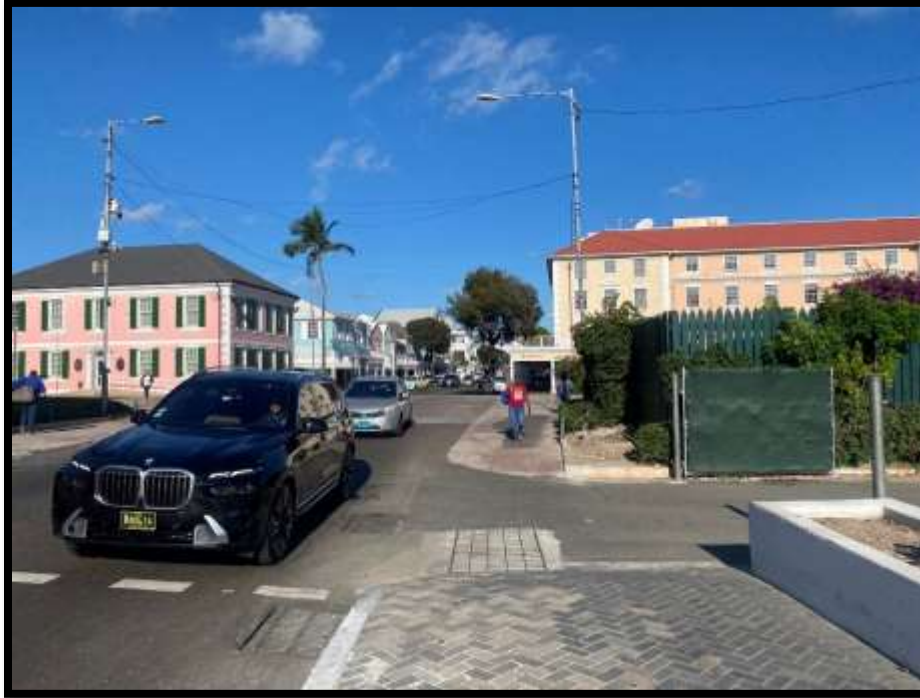
Figure 125. Bay Street with overhead lighting and sewer system and view of Rawson Square Lift Station (green fenced). Source: PlanEHS, 2024.
