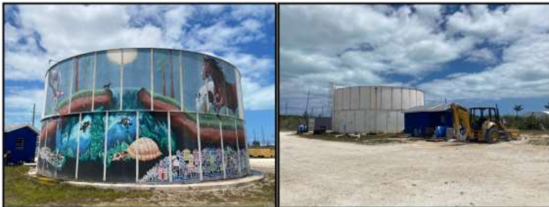
Figure 156. Existing (and damaged) storage tanks at Marsh Harbour Pumping Station. Source: PlanEHS, 2024.
