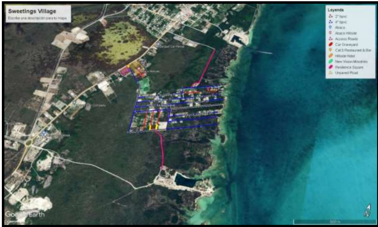
Figure 102. Uncleared and unpaved roads in Sweetings Village (yellow), car graveyard (red) and access roads (pink). Source: PlanEHS, 2024.
