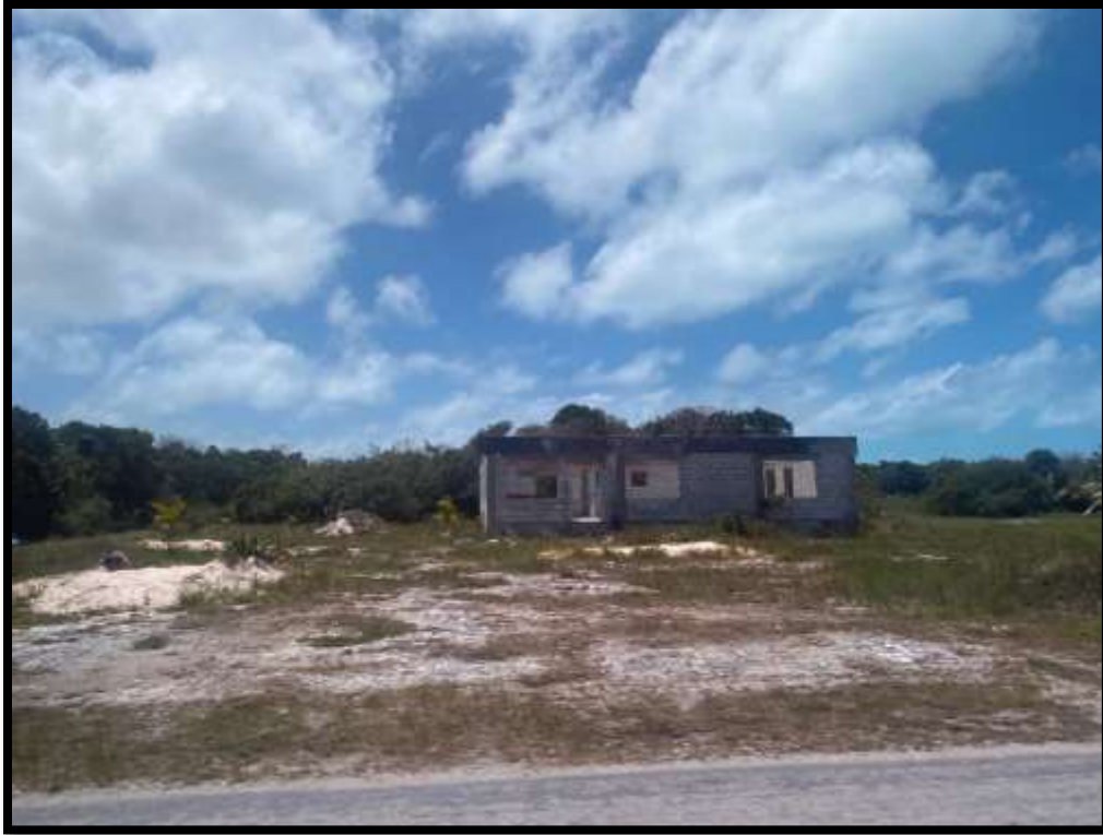
Figure 80. Residential houses in construction along Queen's Highway. Source: PlanEHS
