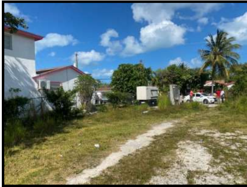
Figure 120. Adjacent residential home of Elizabeth East Lift Station view from unpaved path that leads to Trinidad Way. Source: PlanEHS, 2024.
