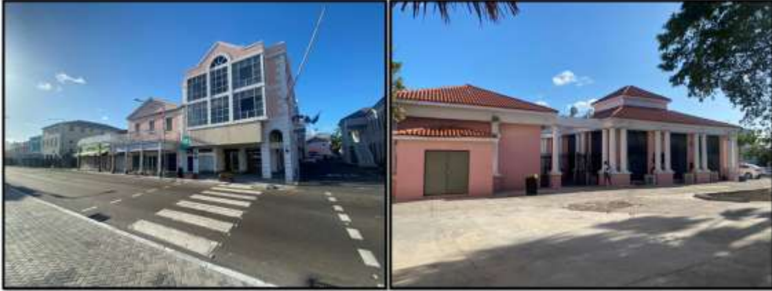
Figure 128. Surrounding buildings from Rawson Square Lift Station. Source: PlanEHS, 2024.
