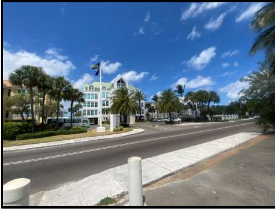
Figure 140. East Bay Street, access to the lift station and resorts located in front of Lift Station. Source: PlanEHS, 2024.
