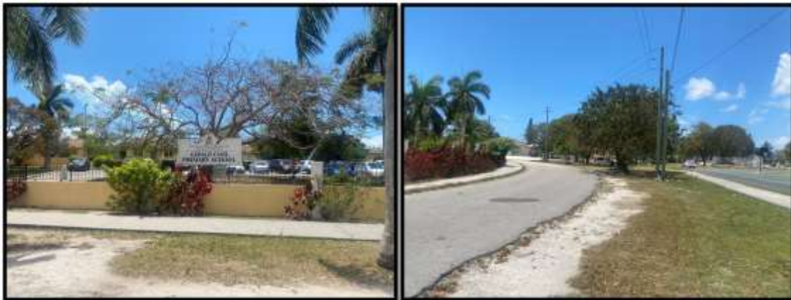
Figure 115. (a) Gerald Cash Primary School, adjacent to Lift Station on Flamingo Gardens Park; (b) Bangladesh Crescent Road. Source: PlanEHS, 2024.
