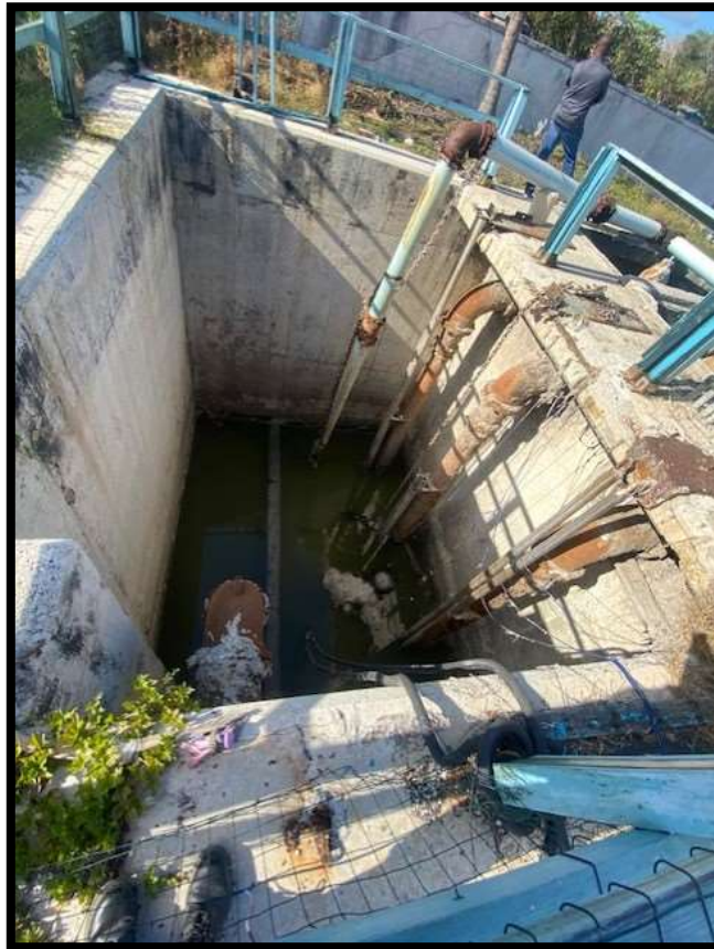
Figure 32. (a) 1 o well chamber and PVC bypass; (b) 2 o well chamber and PVC bypass. Source: PlanEHS
