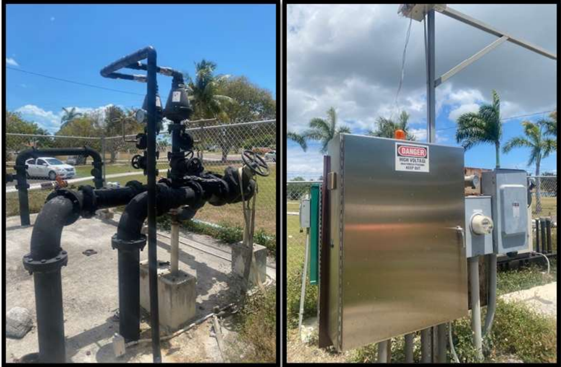
Figure 16. (a) Overground valves; (b) Pump Control Panel. Source: PlanEHS, 2024.
