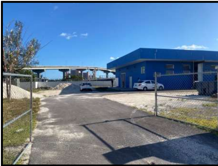
Figure 134. Entrance to Malcolm Park Lift Station, view of the non-operational building and access to Paradise Island on the back. Source: PlanEHS, 2024.
