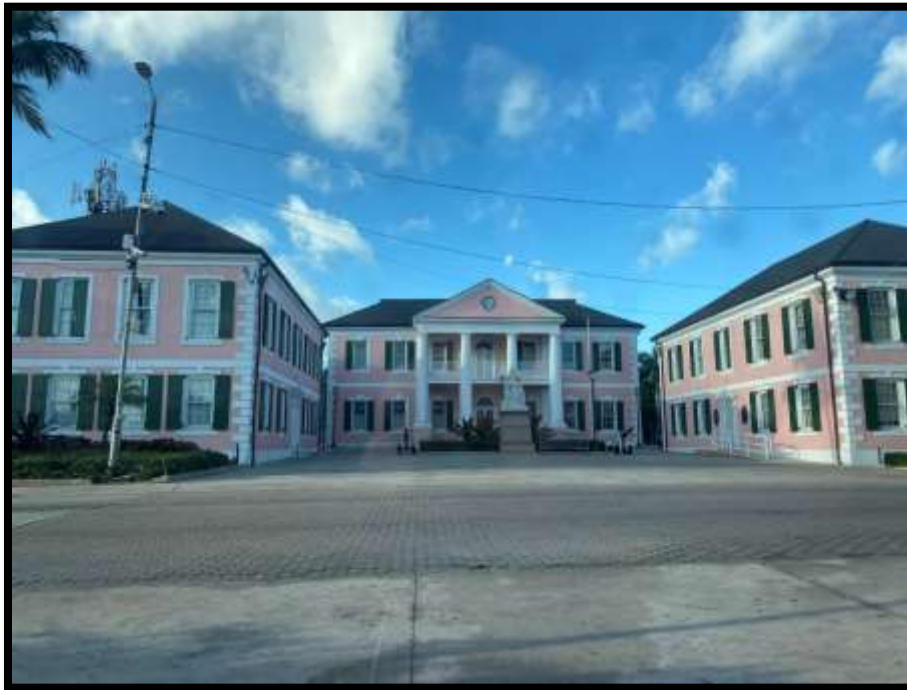
Figure 70. Parliament Square, Historical Buildings located in front of a proposed project site (Rawson Square Lift Station). Source: PlanEHS, 2024.
