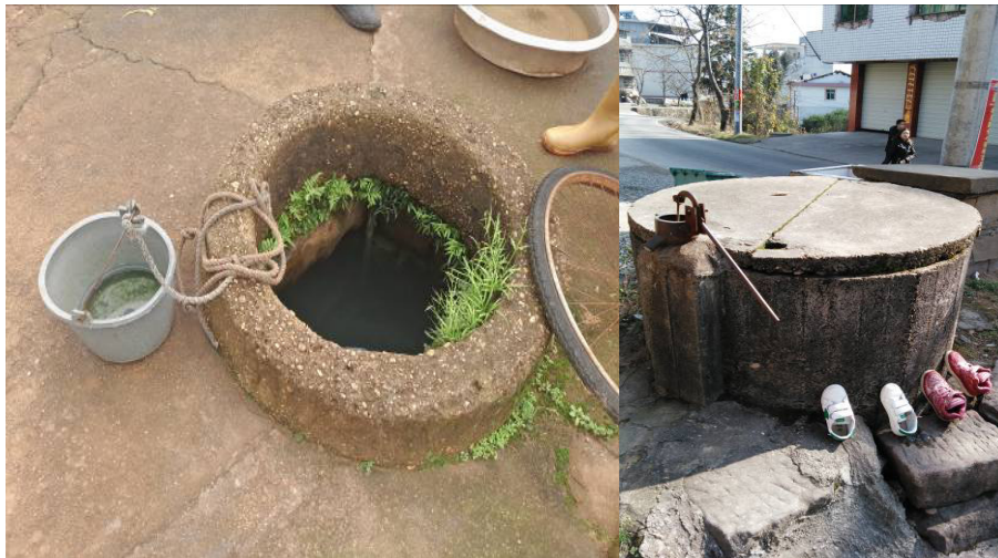
Figure 4-2 Open and pressure wells in use in Dongxiang District and Nanfeng County
