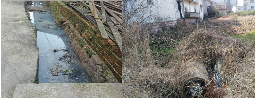
Figure 5-1 Open canal and blind ditch for wastewater discharge
