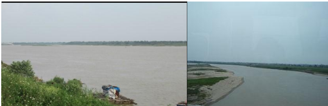
Red River near Ngu Kien and Nguyen Duc pumping stations
