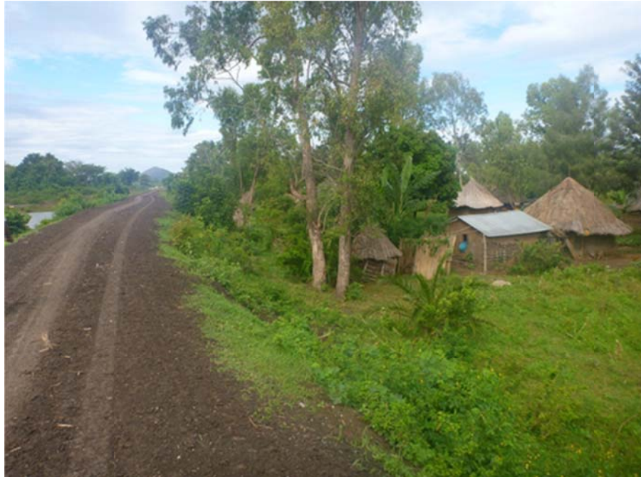
Plate 3: Typical household structures and planted vegetation at the toes of existing dykes. Where these exist, they will be affected by higher and stronger dykes requiring broader base.
