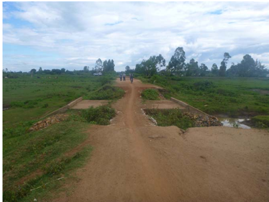
Plate 4: Section of embankment and culverts south of Sigiri boat crossing point. This will be replaced with larger culverts to enhance flow of floodwaters between dykes.
