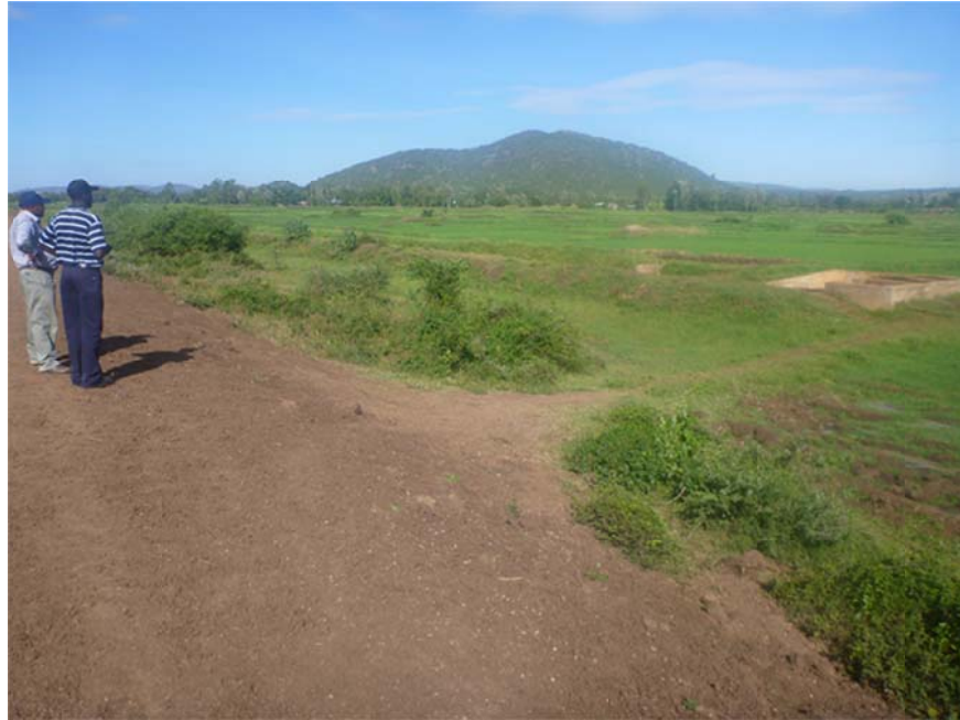
Plate 5: Section of an irrigation canal (RHS) next to the existing northern dyke parts of which may be affected by broadening the dykes.
