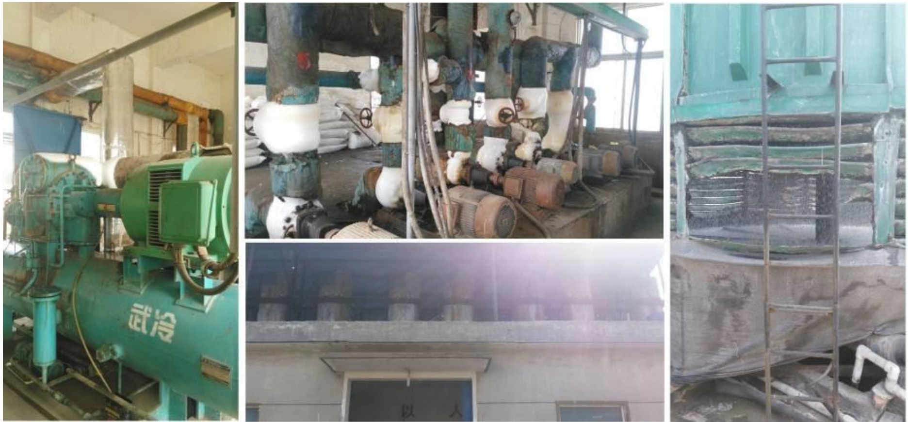
Figure 9 Condensing workshop and condensed water circulation system
