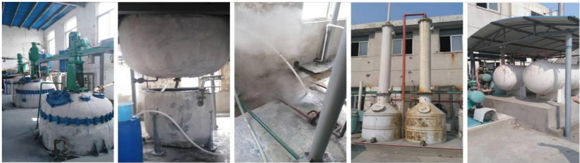
Figure 7 No.1 workshop and hydrogen chloride absorption tower
