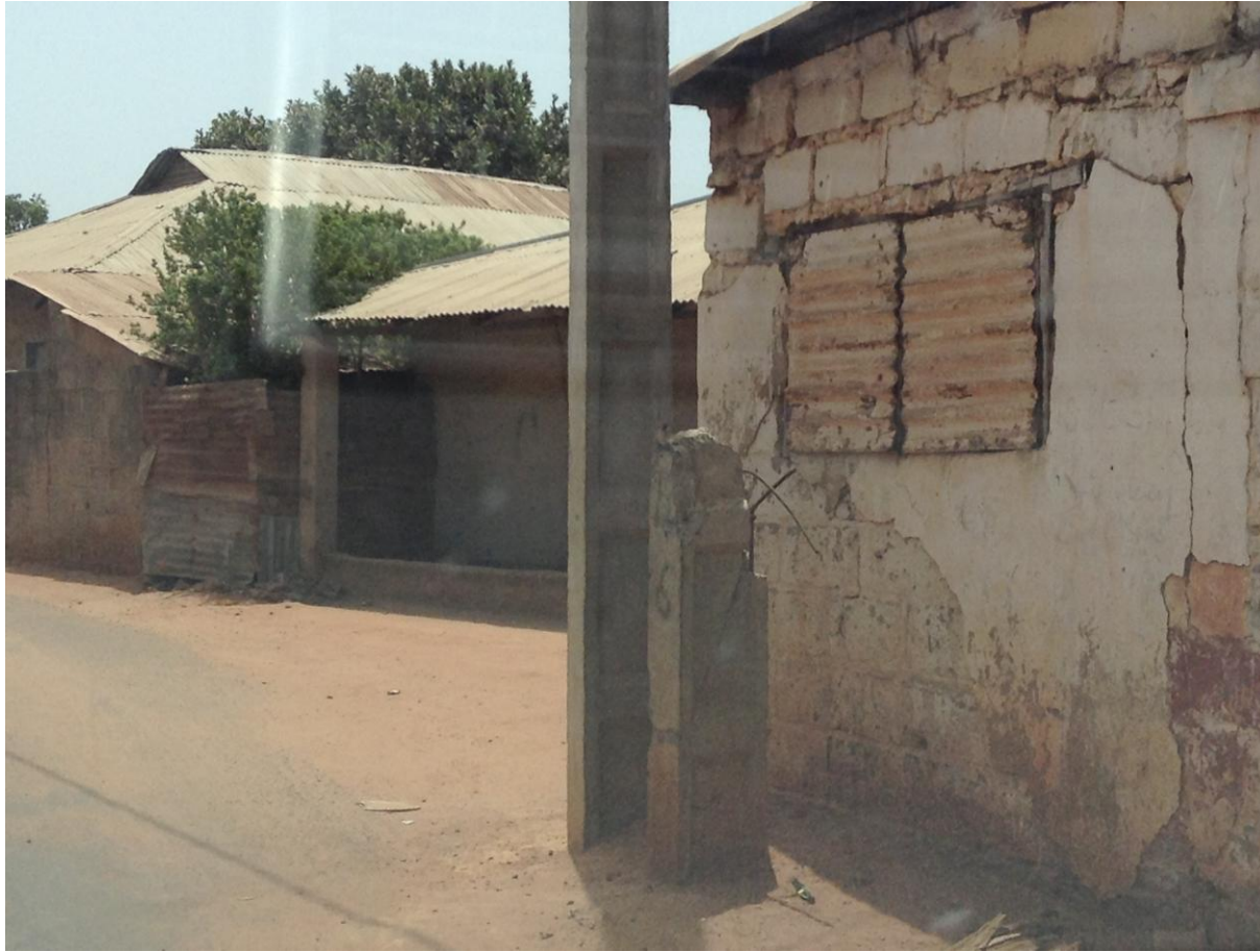
Figure 14: Another disused structure left at site in Brikama
