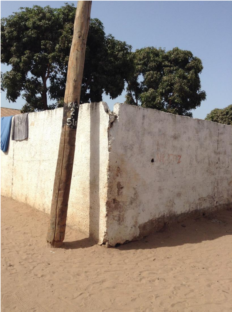
Figure 19 : Existing pole at Wellingerra with evidence of instability at the base
