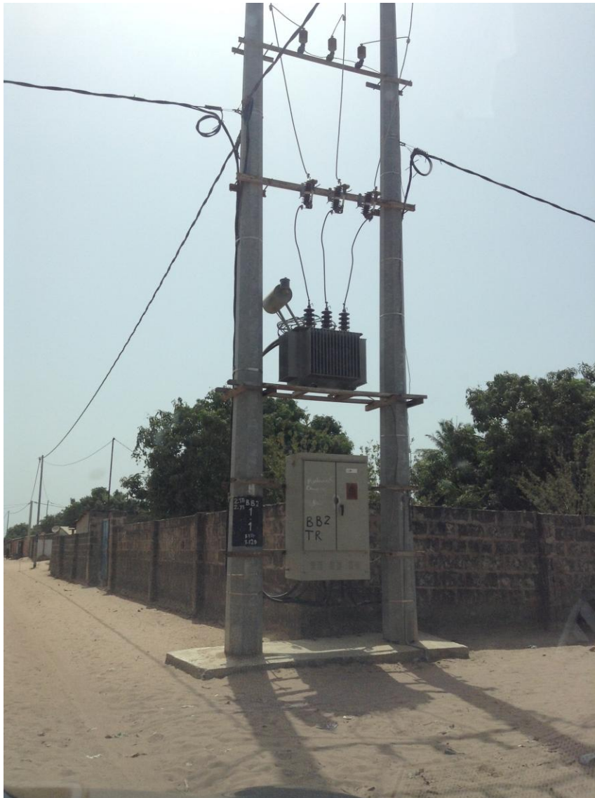
Figure 12: Transformer poles unnecessarily protruding on the road.
