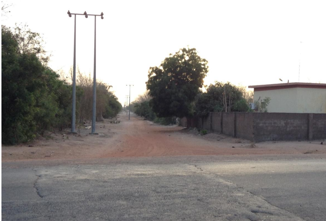
Figure 15: Brikama Medina Substation on the right with road clearance from Nyambia Forest.
