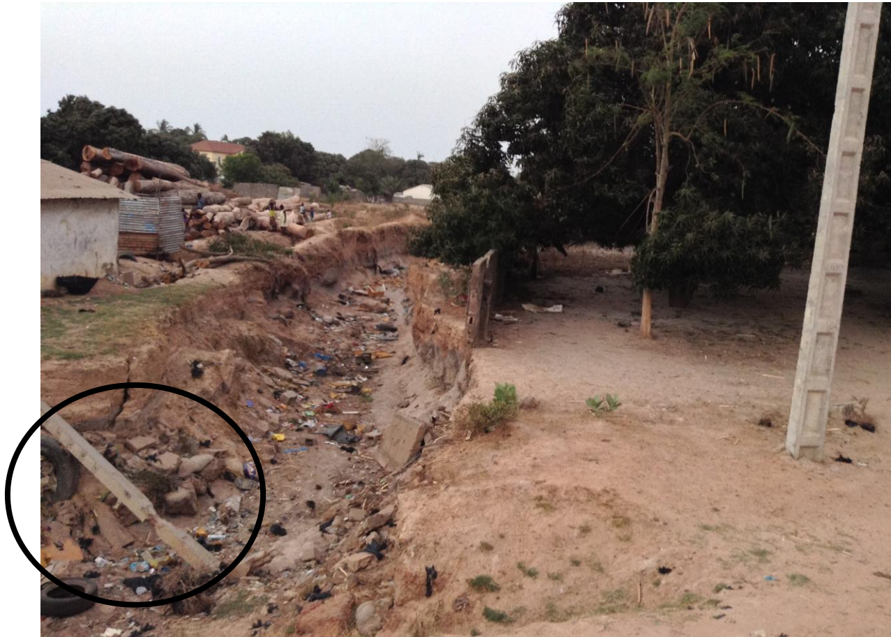
Figure 13: Gully at Abuko Oldfield
