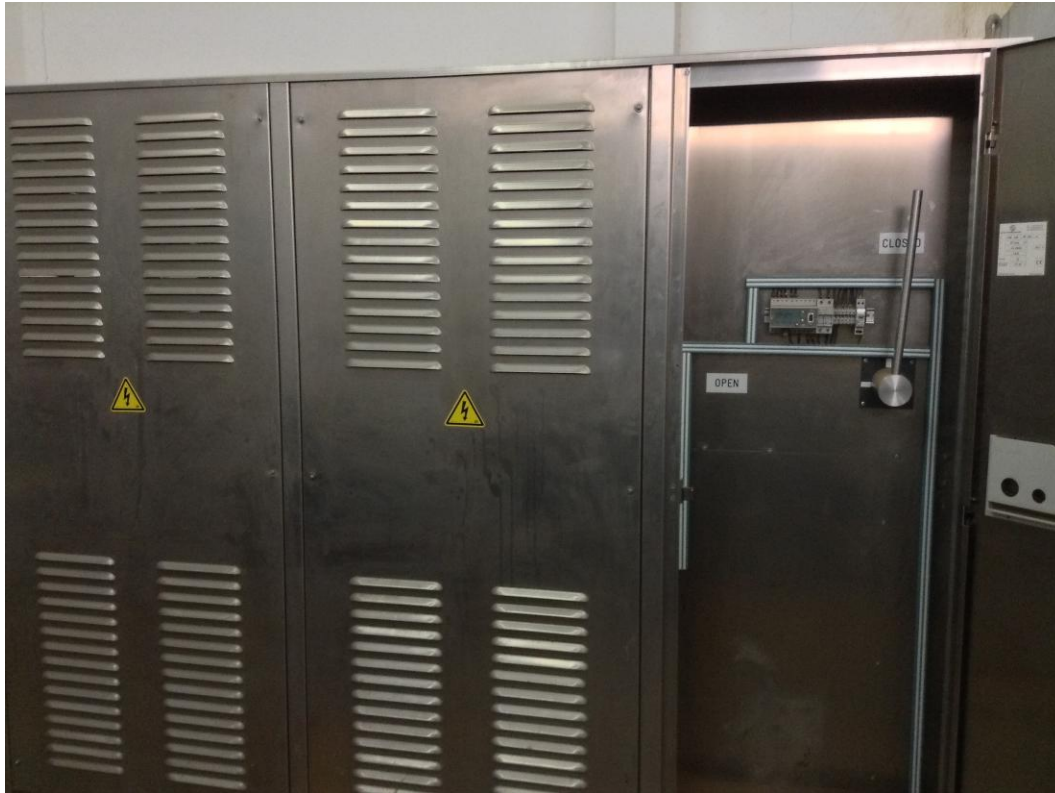
Figure 11: Non-functional capacitor bank at Bijilo Substation.
