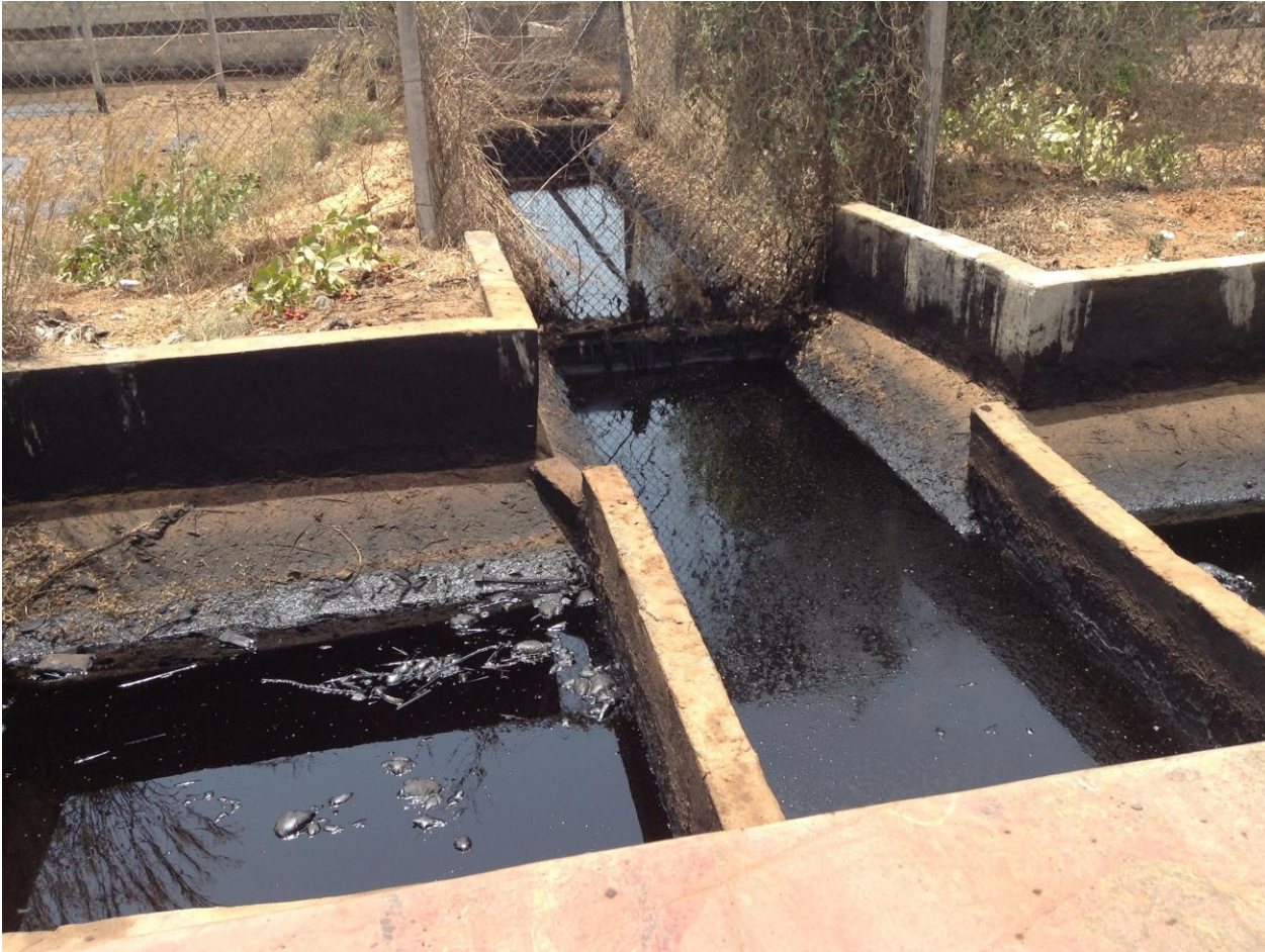
Figure 17: Open drain with sludge oil at Kotu Power Plant
