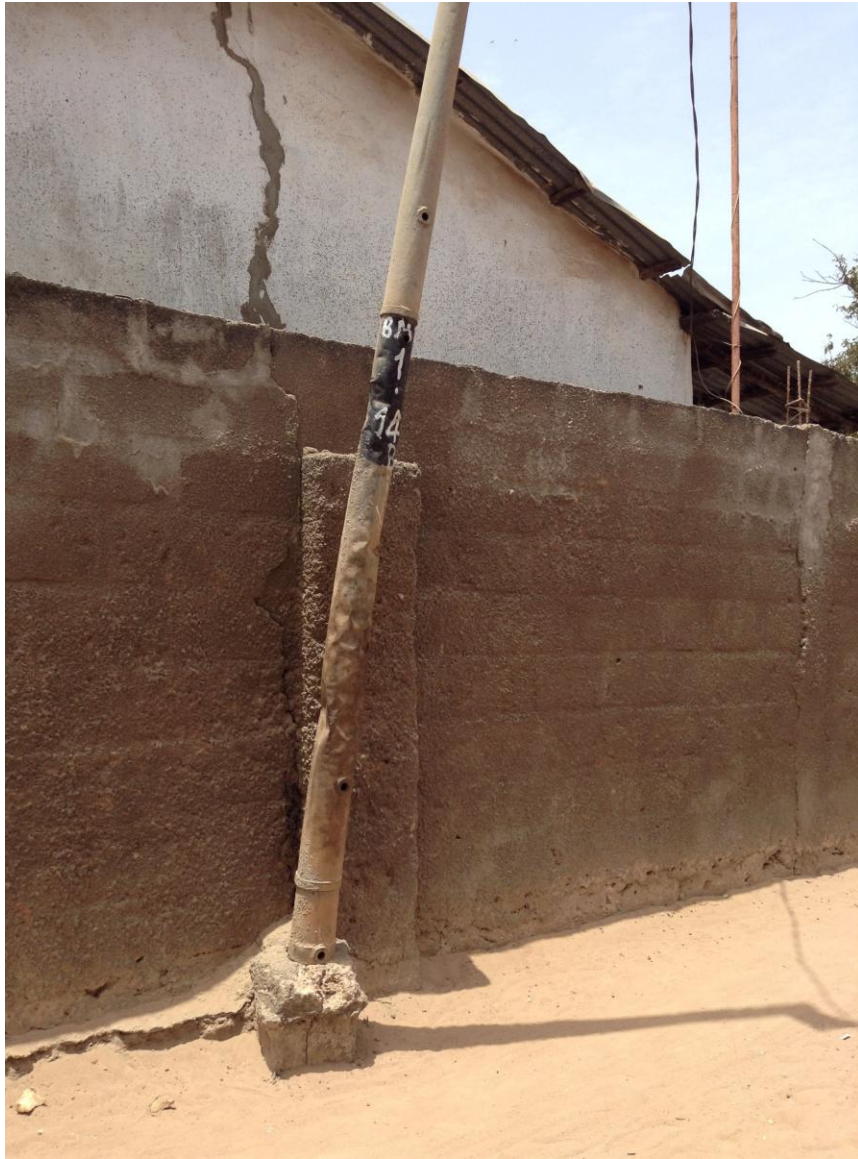
Figure 18: Substandard pole at Brikama
