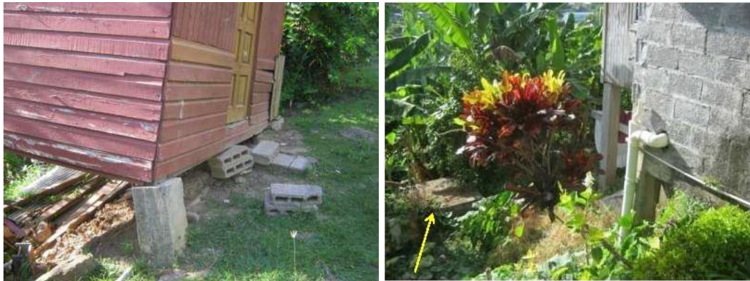
La Sagesse: House foundation issues; septic tank without leach field (top right, arrow)
