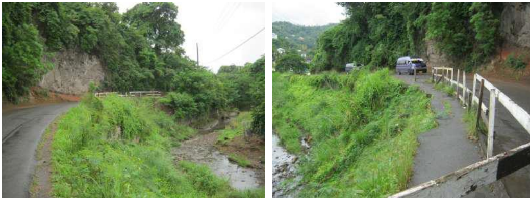
River Road: area of road erosion, river defense failure
