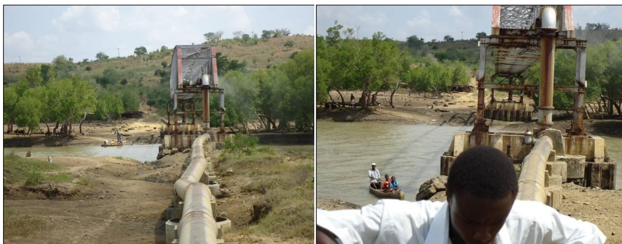
Marere Pipeline crossing towards Mazeras
