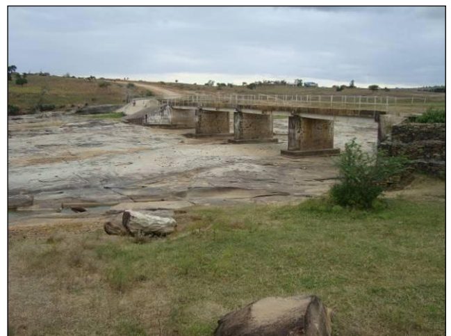
Bridge over Mwache (Mazeras – Kinango)
