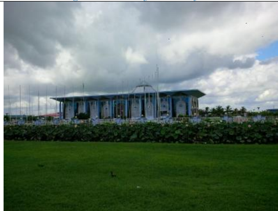
Picture 8: Southern Canal in front of the Authur Chung Convention Centre in the Background. The tertiary drains will flow into this canal
