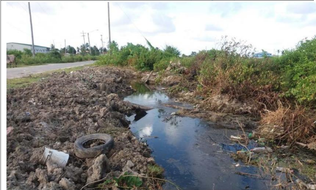
Picture 1: Existing ditch that borders the western side of the Proposed Project Site
