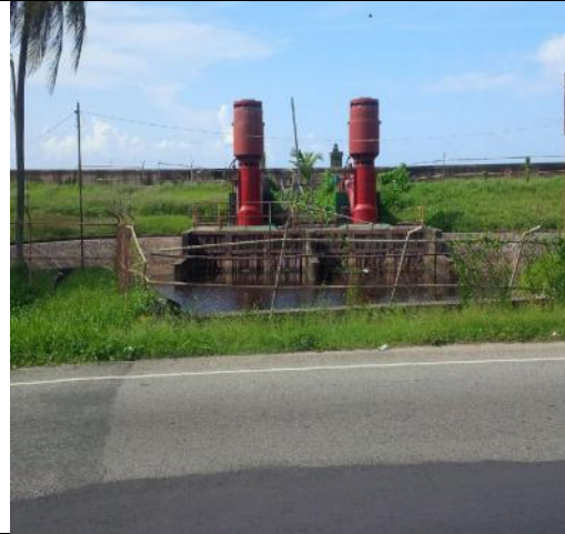
Picture 3: The Liliendaal Pumps that services the Project Area
