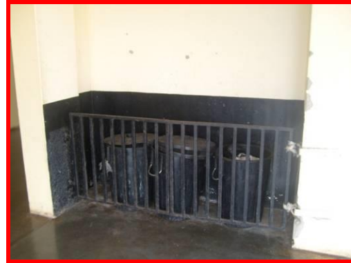
Figure 7-1 Temporary storage for waste
