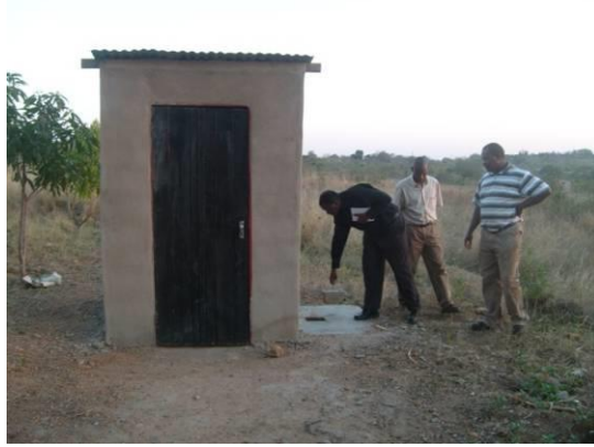
Pit with Pit Latrine for home based care
