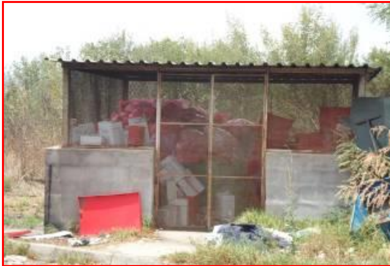
Figure 7-2 Example of a centralized storage.
