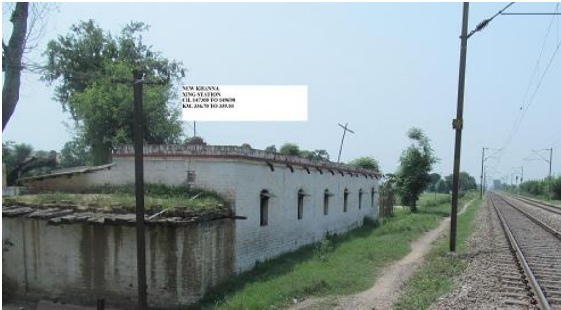
Figure 2.8: Site for New Khanna Crossing Station
