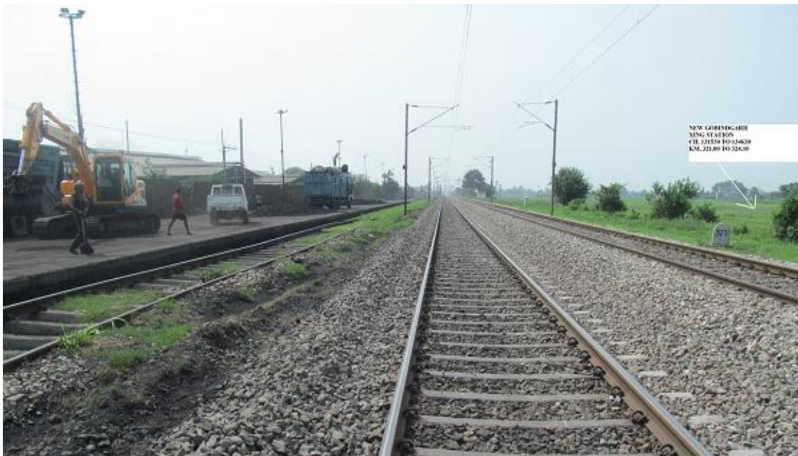
Figure 2.9 : Site for New Govindgarh Crossing Station
