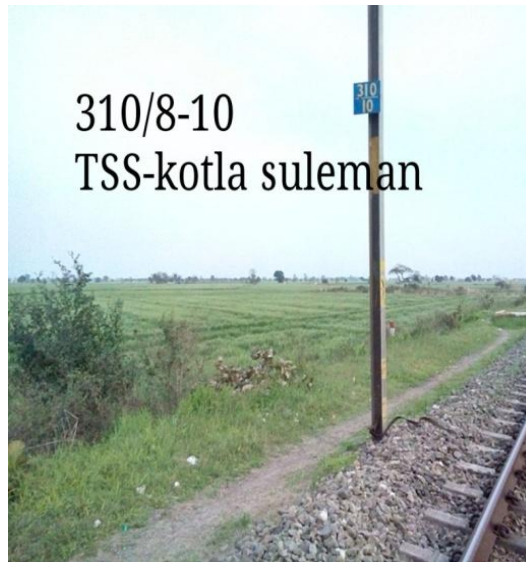
TSS-Kotla Suleman- km 310/8-10
