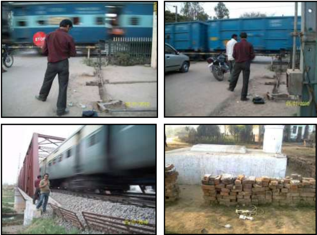
Vibration Monitoring Along the Alignment
