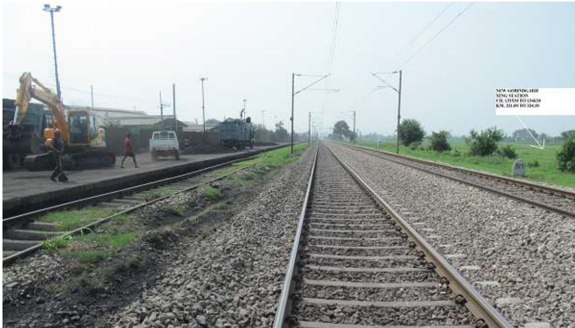
Figure 2.9 : Site for New Govindgarh Crossing Station
