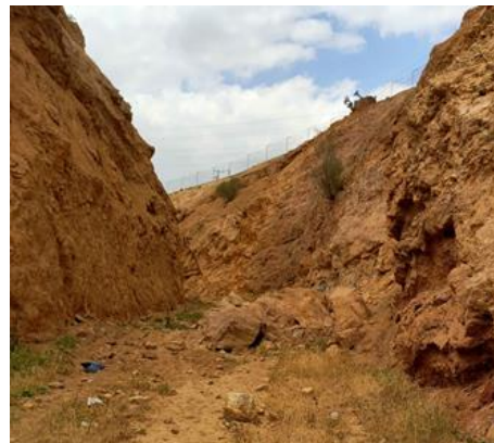
Photo 2: Instable cut and Rock Falls (weir to stelling basin)
