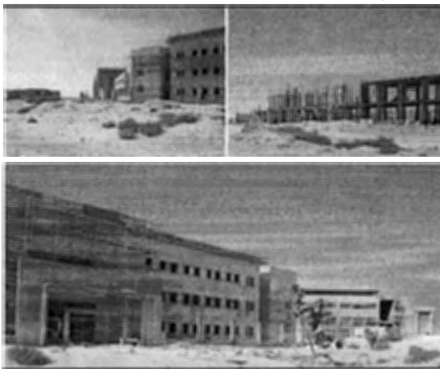
Figure 3.7 Pictures of the current University of Nouakchott Construction Site (November 2012)
