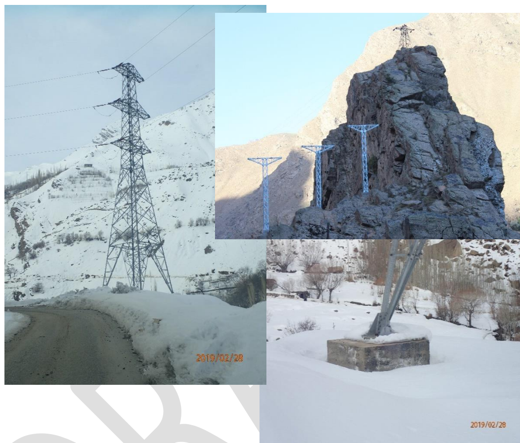
Figure 4. Examples of towers: angle tower at left, three suspension poles on uneven terrain at top right, and example of foundation at lower right
