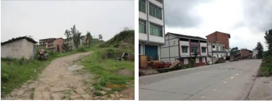
Figure 3.4.3-1 Status Quo of Construction Access Road
