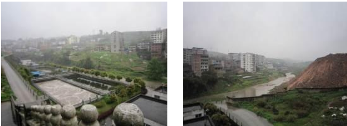
Figure 5.3.7-1 Status Quo of Linshui No. 1 WWTP
