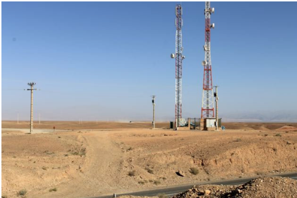
Plate 15-1 Communication towers at the intersection of N10 and the site access road
