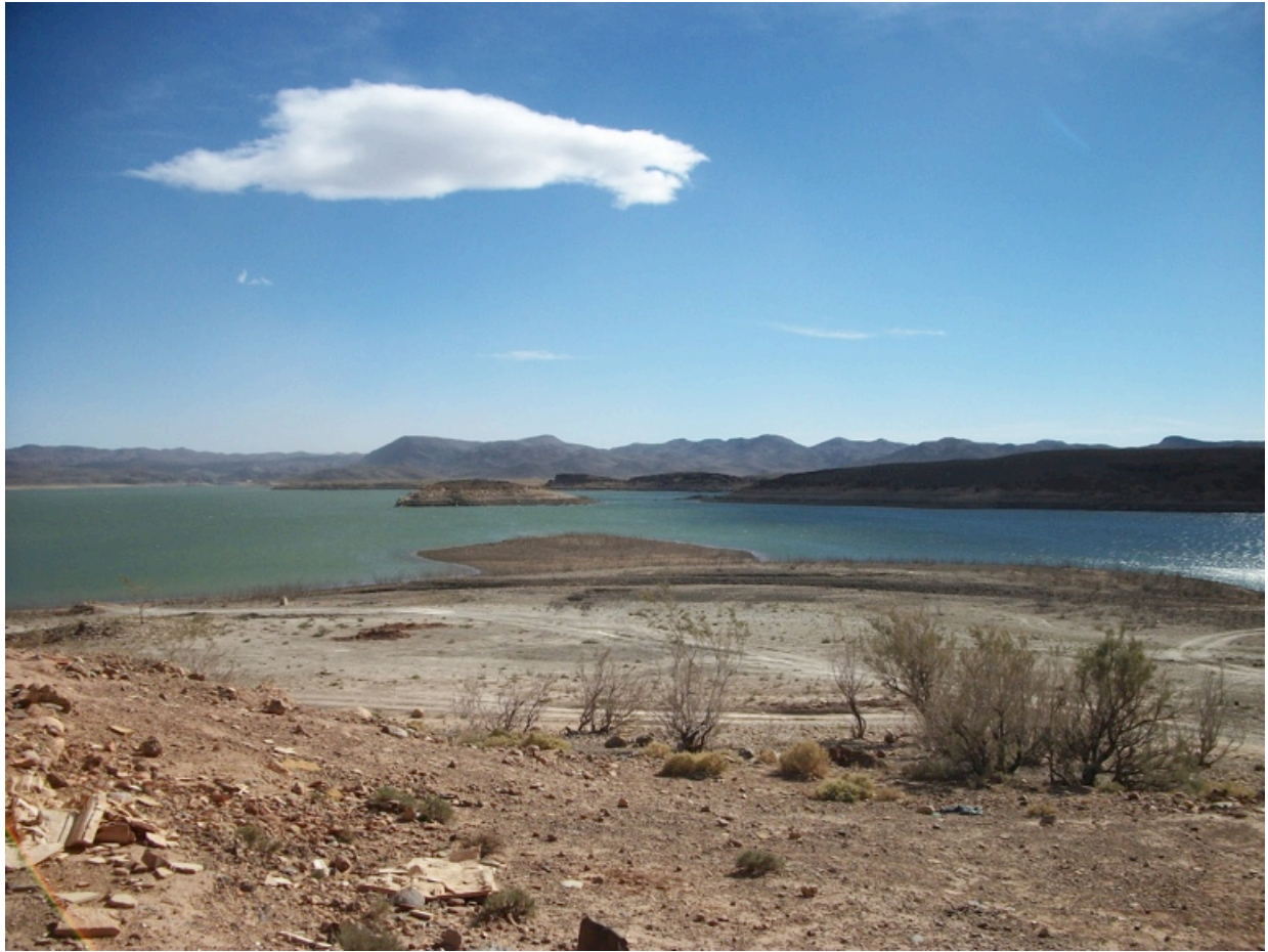
Plate 3-8 Mansour Ed Dahbi Reservoir
