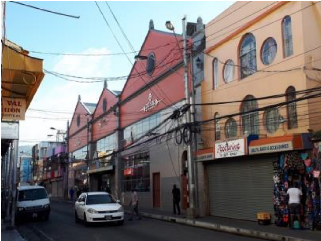
Charlotte street façade
