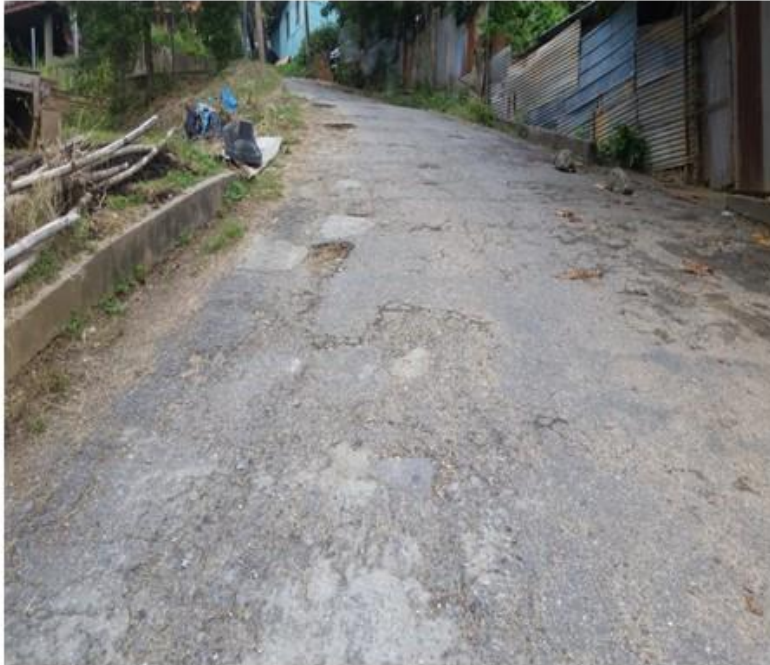
Cracks, potholes and breaking away throughout the main road
