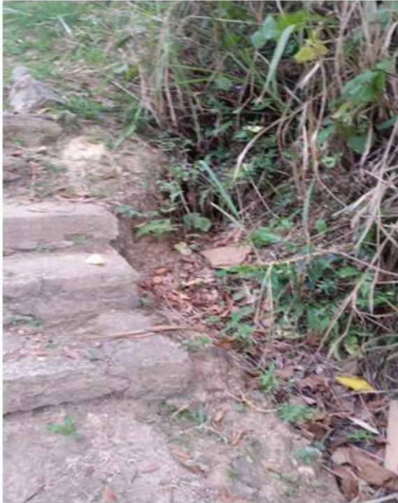
This stair way was constructed by residence many years ago but a drain was naturally formed from the rainfall.
