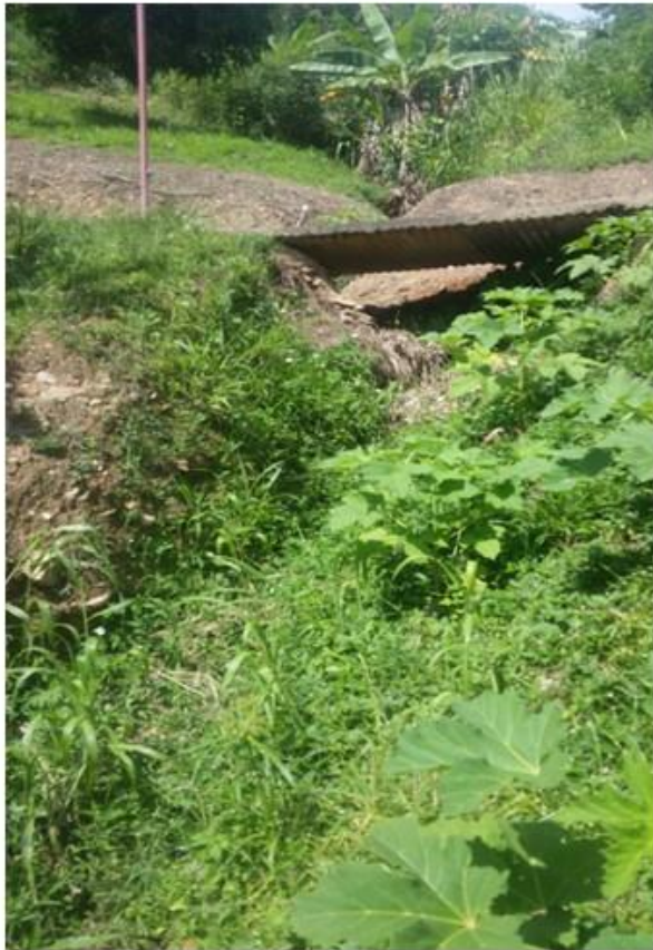
This bridge was made by residence As seen it is poorly made and can Collapse and anytime as a natural River has formed below it.
