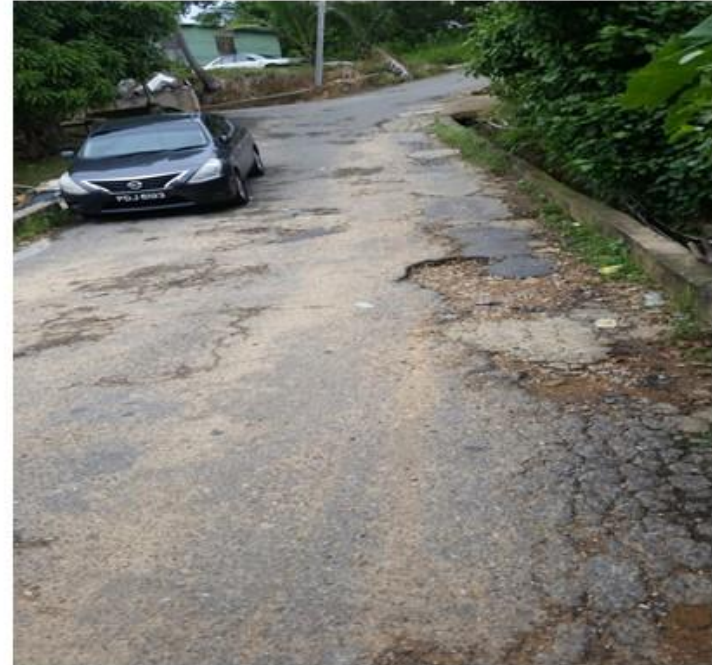
Cracks, potholes and breaking away throughout the main road
