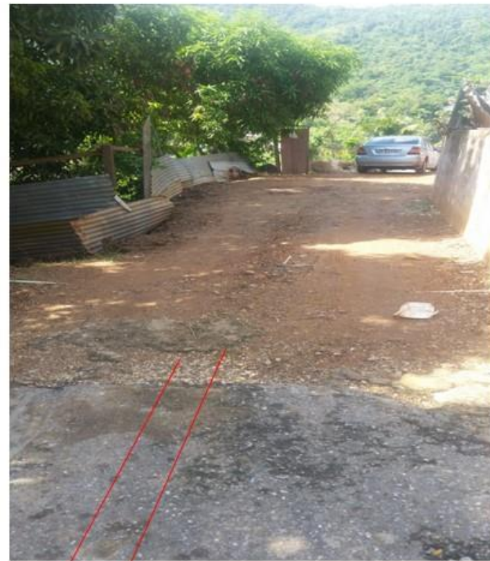
Pitch material breaking away due to rainfall and lack of proper drains
