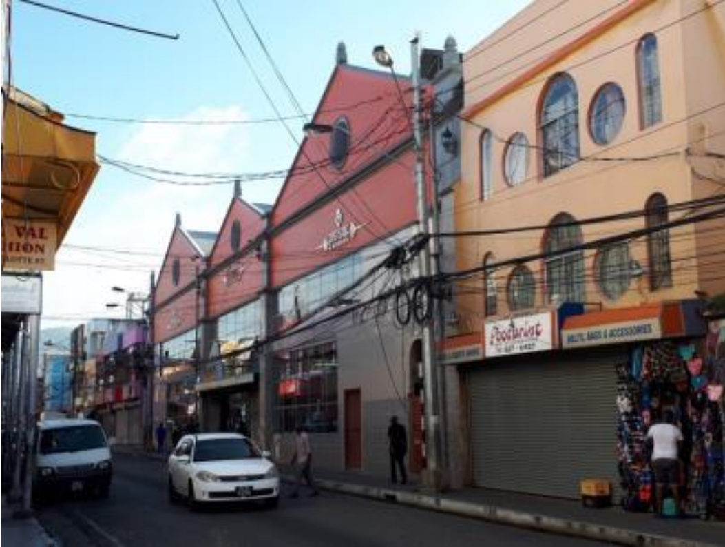
Charlotte street façade
