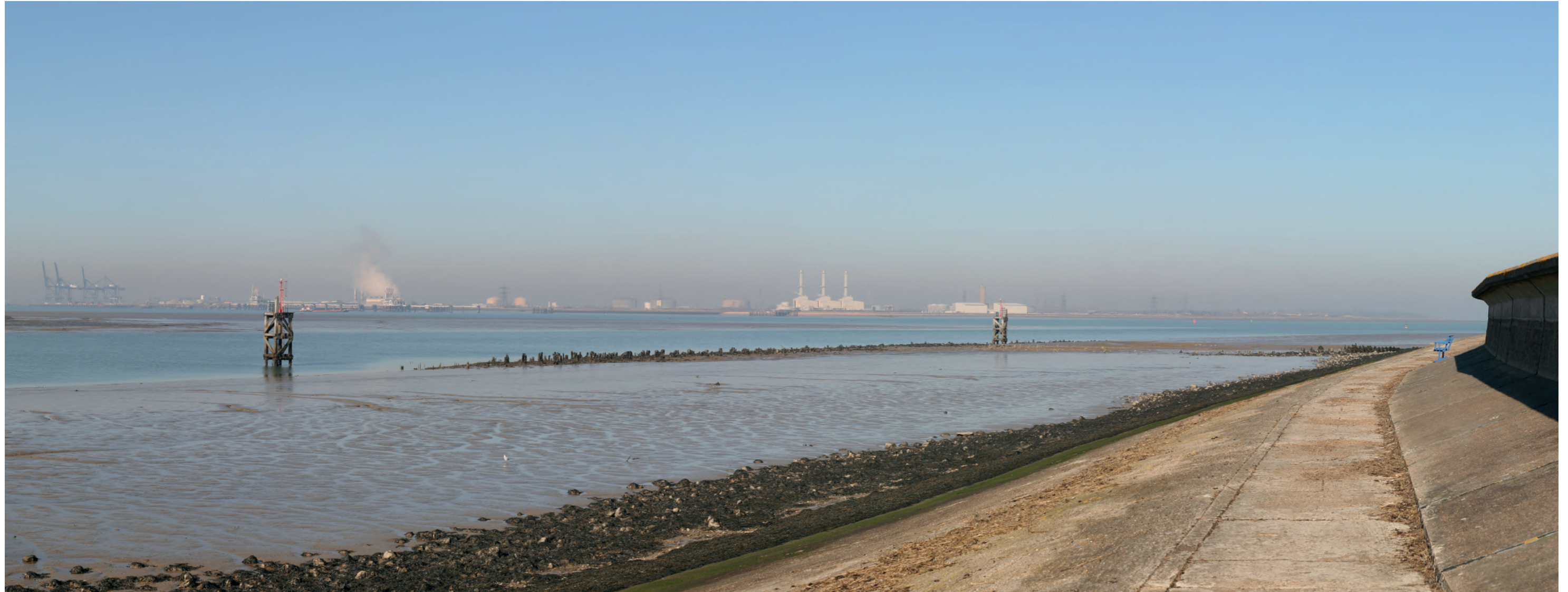
Figure: 5.14a Viewpoint 7 - Queenborough Coastal Path Existing View
