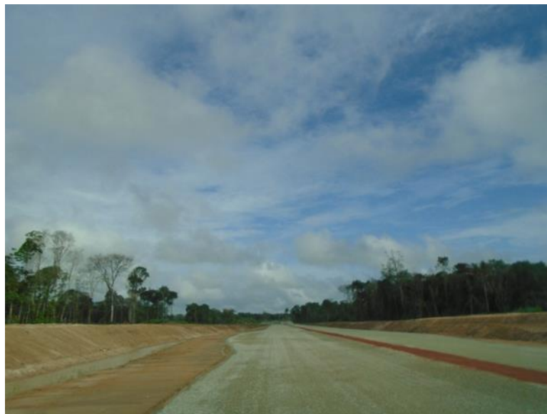
Figure 6: The Afobaka Road-JFK Highway connection road under construction
