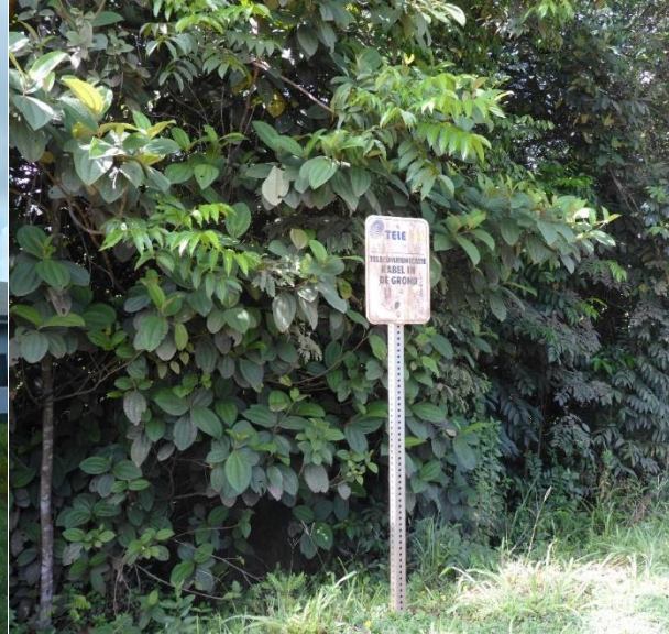
Telesur underground cable along the Brownsweg
