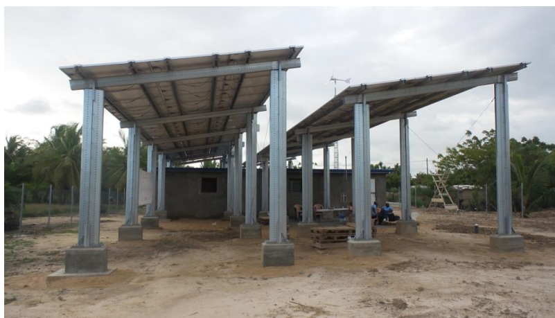
Figure 10: Technical building with a pergola (Source: TTA)
