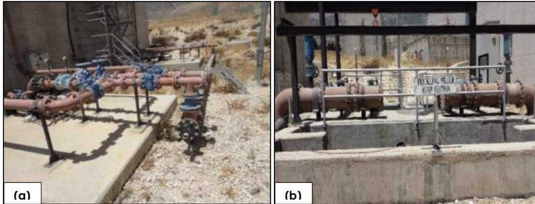
Figure 3-1 Pump stations for digester tanks (a) and Tricking Filter Unit (b)
