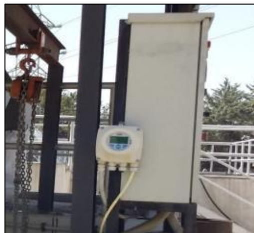
Figure 3-3 Influent Flow Meter
