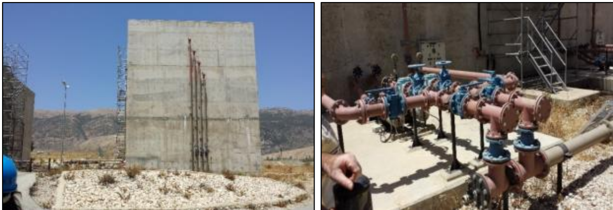
Figure 3-9 Digester tank and its pump station
