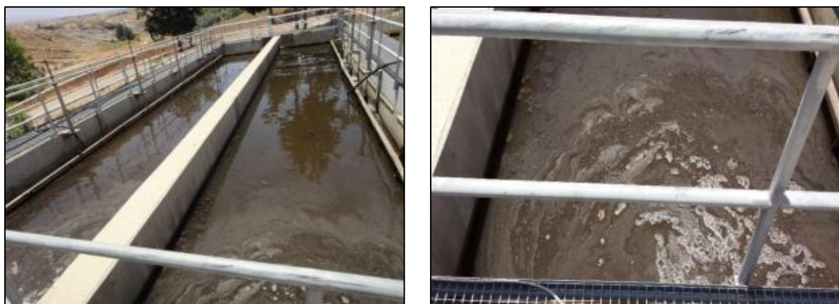
Figure 3-7 Secondary or Final Clarifier showing sudsy, billowing and bulking sludge
