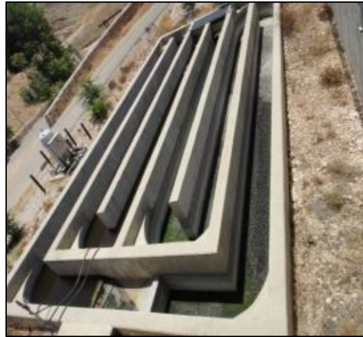
Figure 3-8 Chlorine Contact Tank
