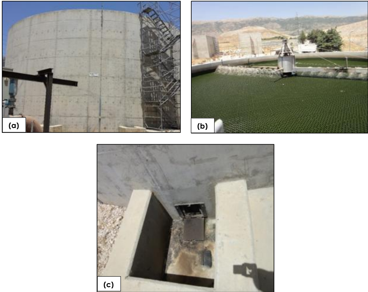
Figure 3-6 Trickling Filter Unit showing the main TF building (a) and the rotation of distribution arms (b) and Ventilation door (c)
