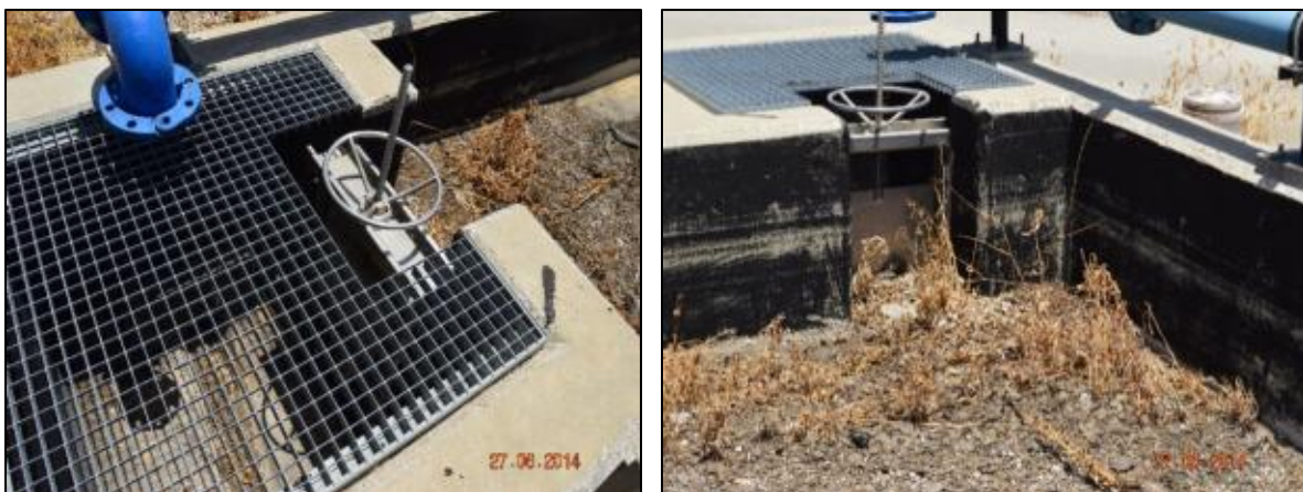
Figure 3-10 Supernatant evacuation system of the sludge: slucice gates
