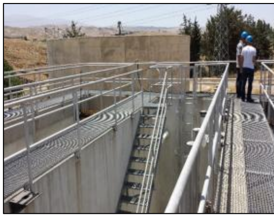
Figure 3-12 Safe Catwalk and Ladders
