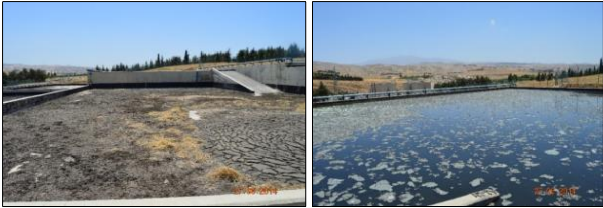
Figure 3-11 Sludge drying lagoons showing sludge cakes and vegetation
