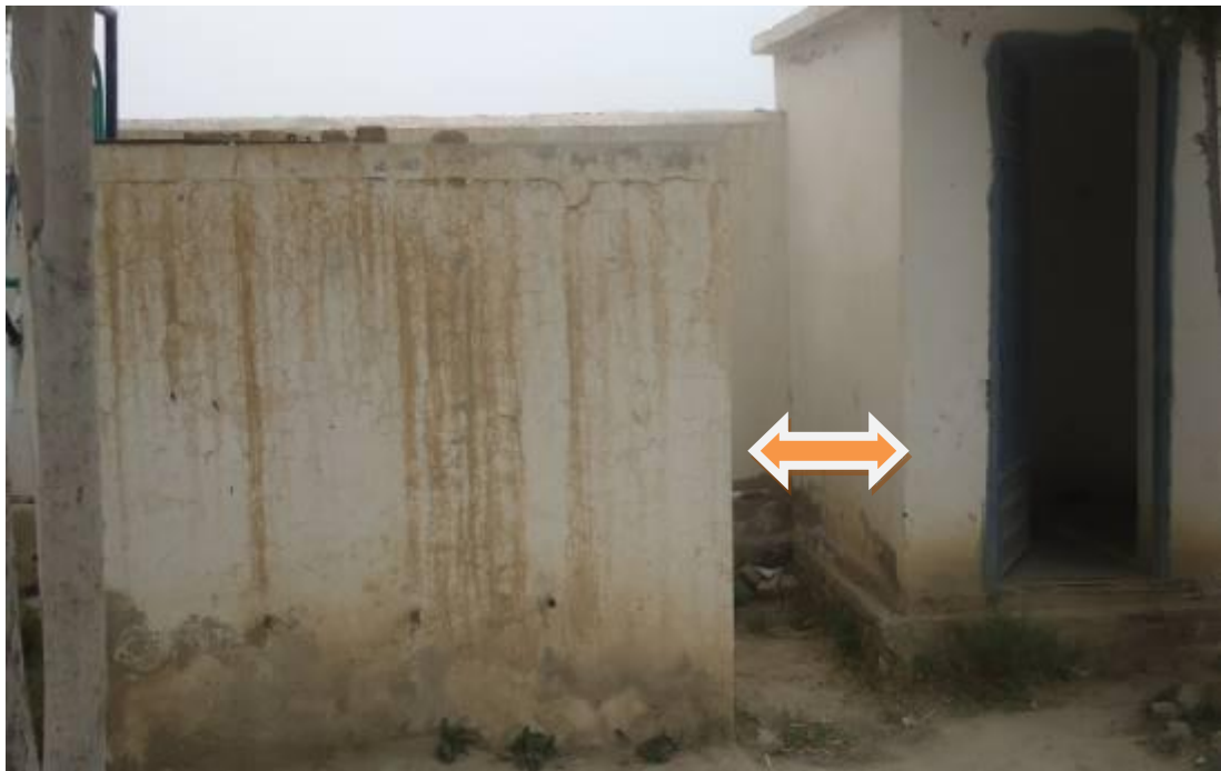
Figure-24: GGPS Baharwala, District Killa Saifullah (water storage tank and laterine)
