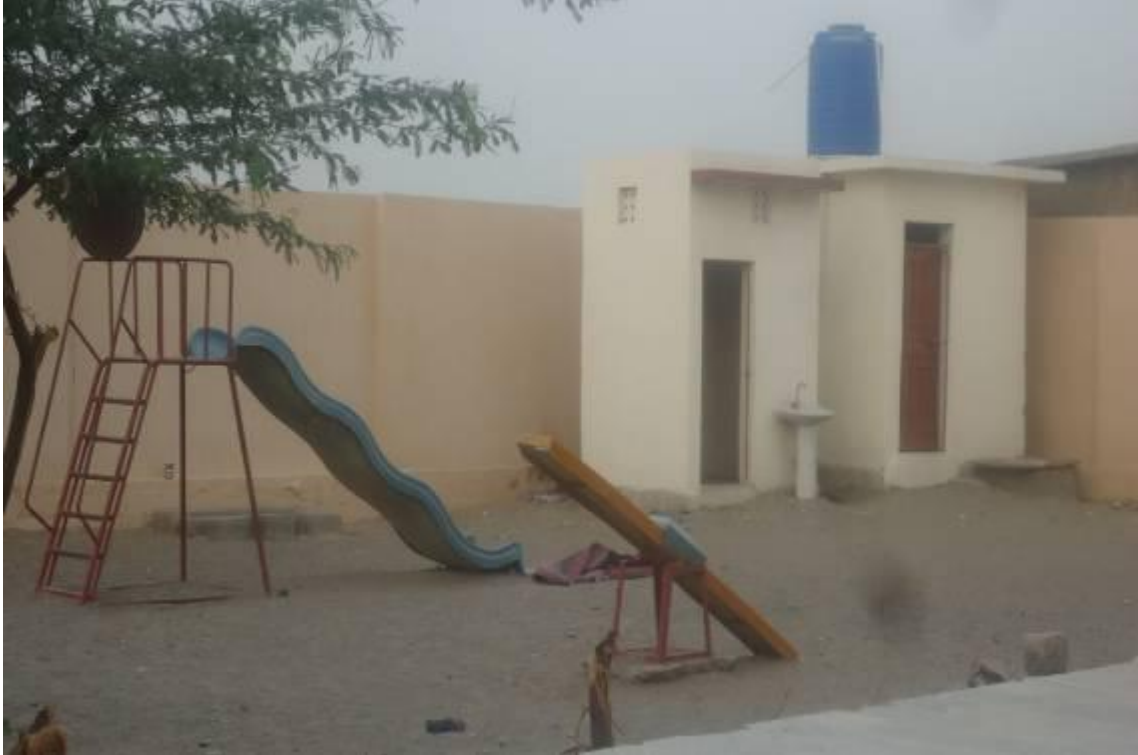
Figure-17: Overview of newly constructed GGPS Morand Colony Uthal, District, Lasbela
