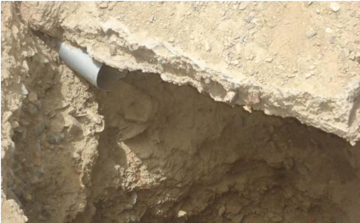
Figure-20: GGPS/Bandat Amandzai, District Killasaifullah (damage sokage pit of latrine)
