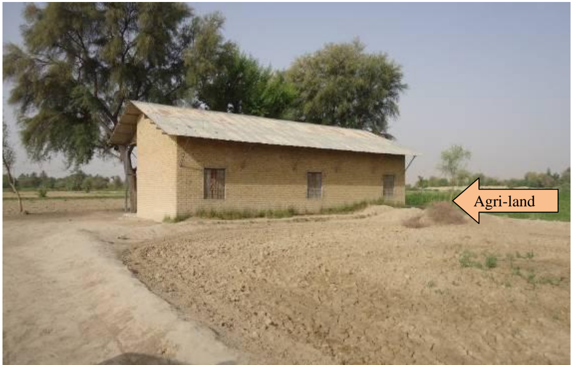
Figure-27: GBPS/Faiz Abad (without latrine and boundary wall), Kachhi District
