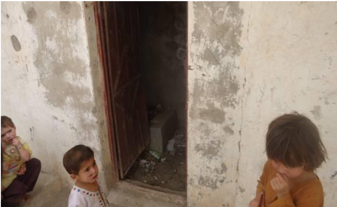
Figure-22: GBPS/Shabozai, District Killasaifullah (un-hygienic latrine without water connection)
