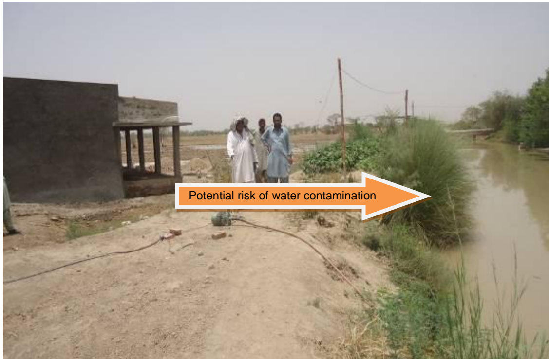
Figure-32: GGPS /Nasrullah Rind, UC-4, District, Jaffer Abad (under construction)
