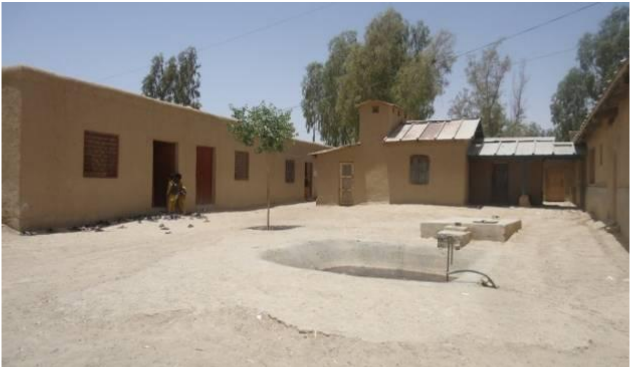
Figure-6: Water Storage Facility in GBMS Cant Loralai bazaar
