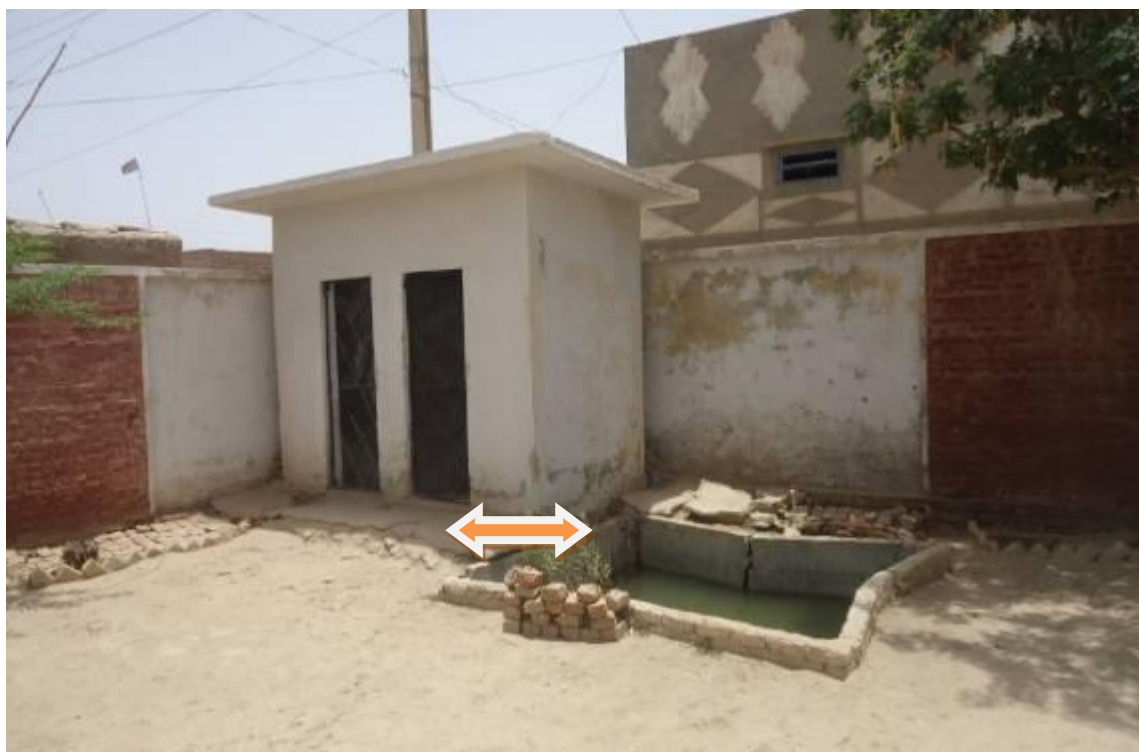
Figure-34: Latrine close to Water Storage Tank (GGPS Shaeed Murad Colony, District Jaffer Abad)
