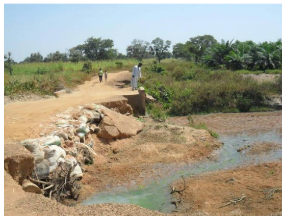
Plate 1.36: Wukari Road Junction – Mayo Reneyow Road, Taraba State
