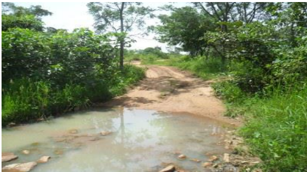
Plate 1.29: Alakolo Stream Across Oke-Oyi – Jokolu Road, Kwara State.
