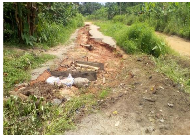
Plate 1.2: At Bende – Ntalakwu Road, Abia State.
