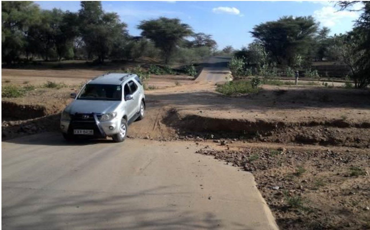
Plate 2: Soil Erosion covering one of the drifts
