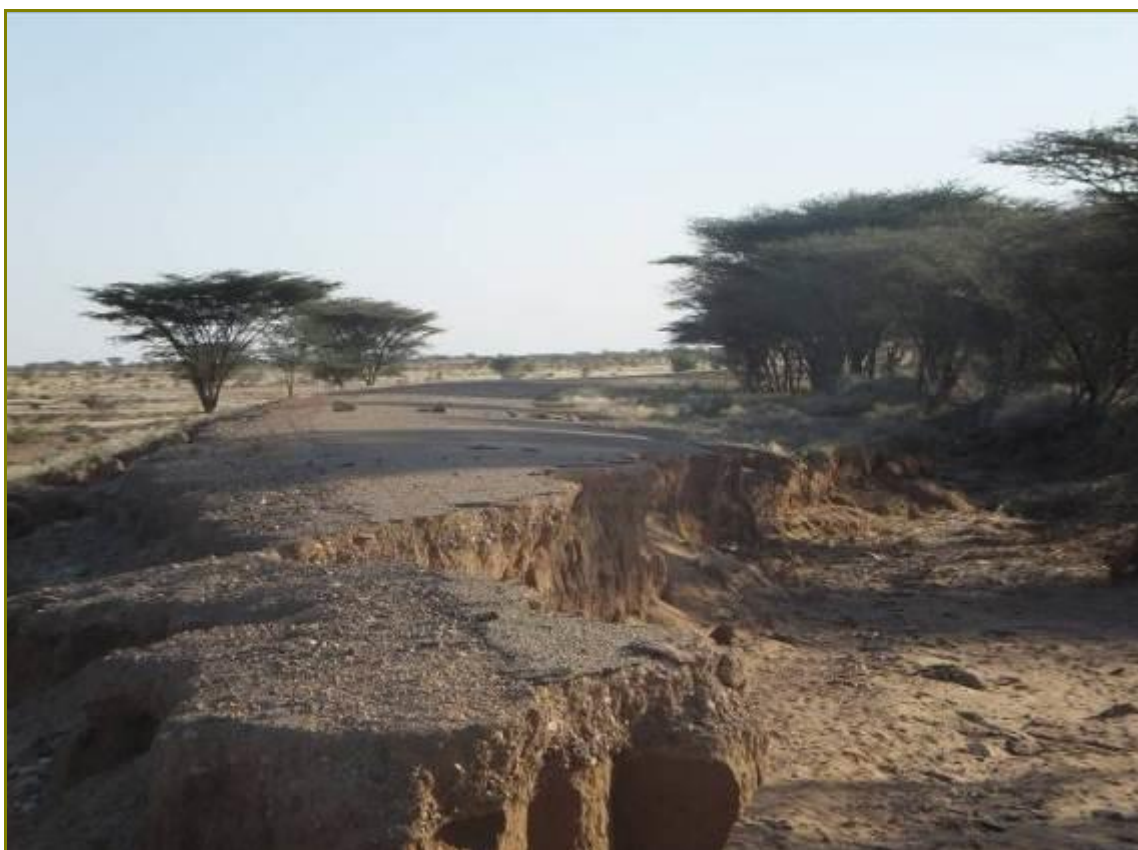
Plate 20: An eroded road embankment along the Lodwar - Kalokol Road
