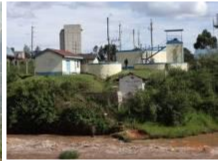
Water Supply at Mois Bridge
