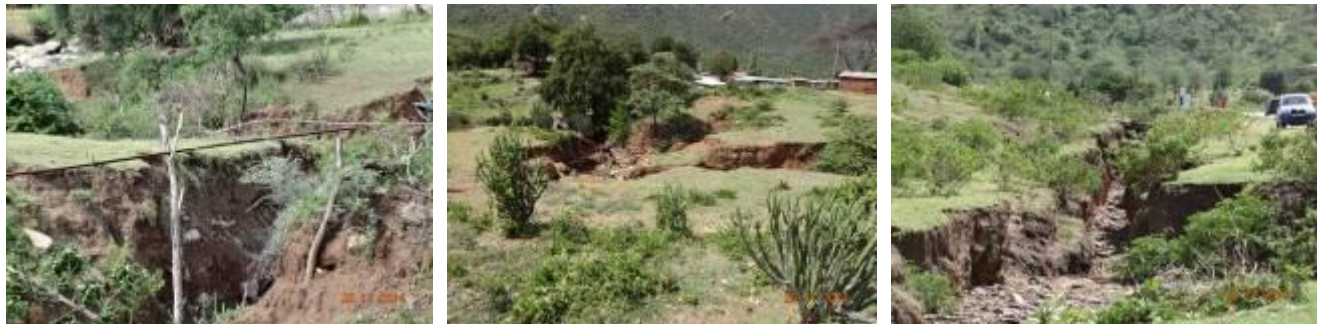
Eroded Spots Associated with Drainage at Culvert Outfalls (Typical of Km96+000 – Km164+000)
