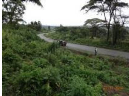
Road Safety Black Spot at ~Km88+000
