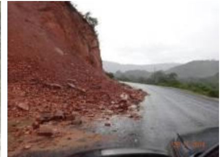
Landslide in Kamatira Forest Edges
