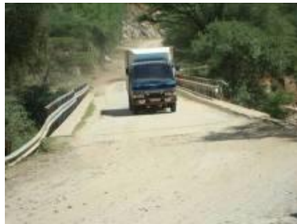
Bridge Over Moruny River
