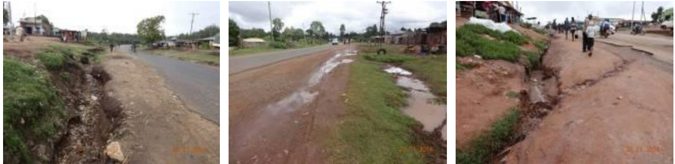
Compromised Roadside Drainage (Typical of KM0+000 – Km96+000)
