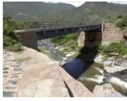
Kopro River Bridge
