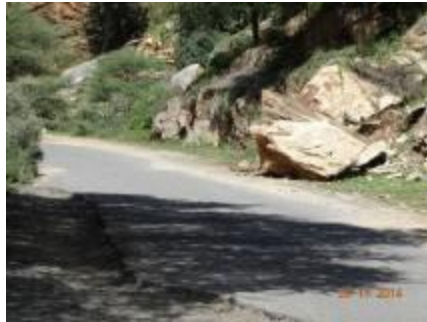
Falling Rocks at Marich Pass
