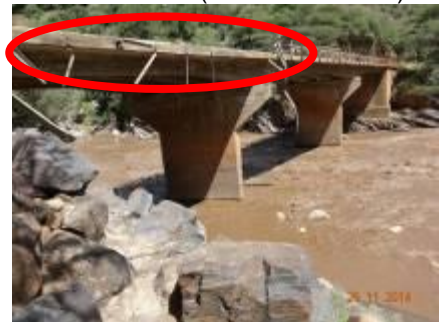
Risks from Bridges (Muruny River Bridge)
