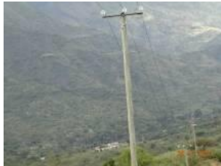
Power Transmission Line
