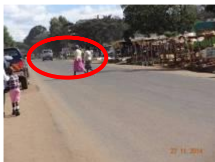
Road Safety Risks at Mois Bridge
