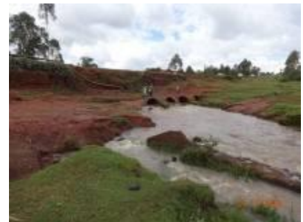
Kipsaina River Bridge
