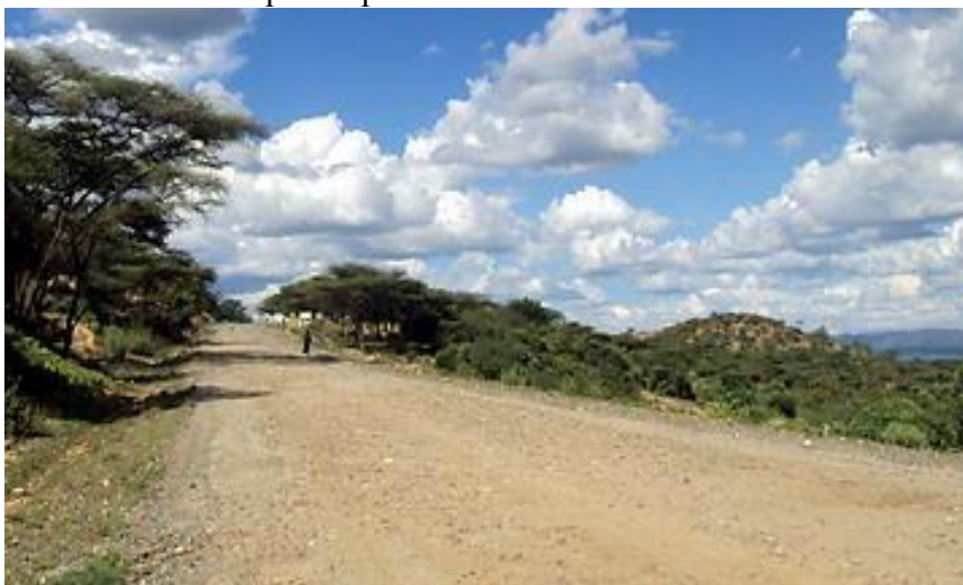
Figure 3-2: Existing Condition of Project Road on Section near Marich Pass
