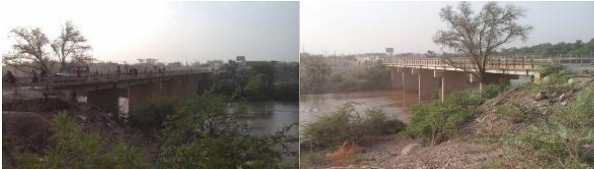
Figure 3-6: Condition of existing bridge at Lodwar– Not wide enough, only one lane
