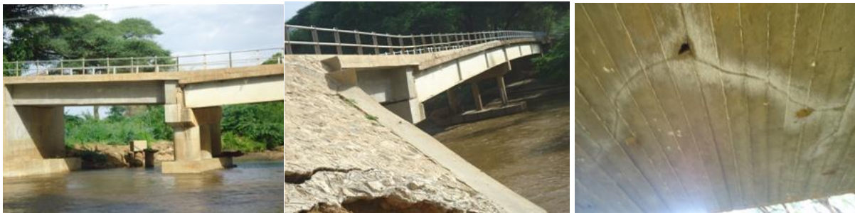
Figure 3-5: Condition of existing bridge at Kainuk – deflection, cracks and ingress of water underneath the slab deck
