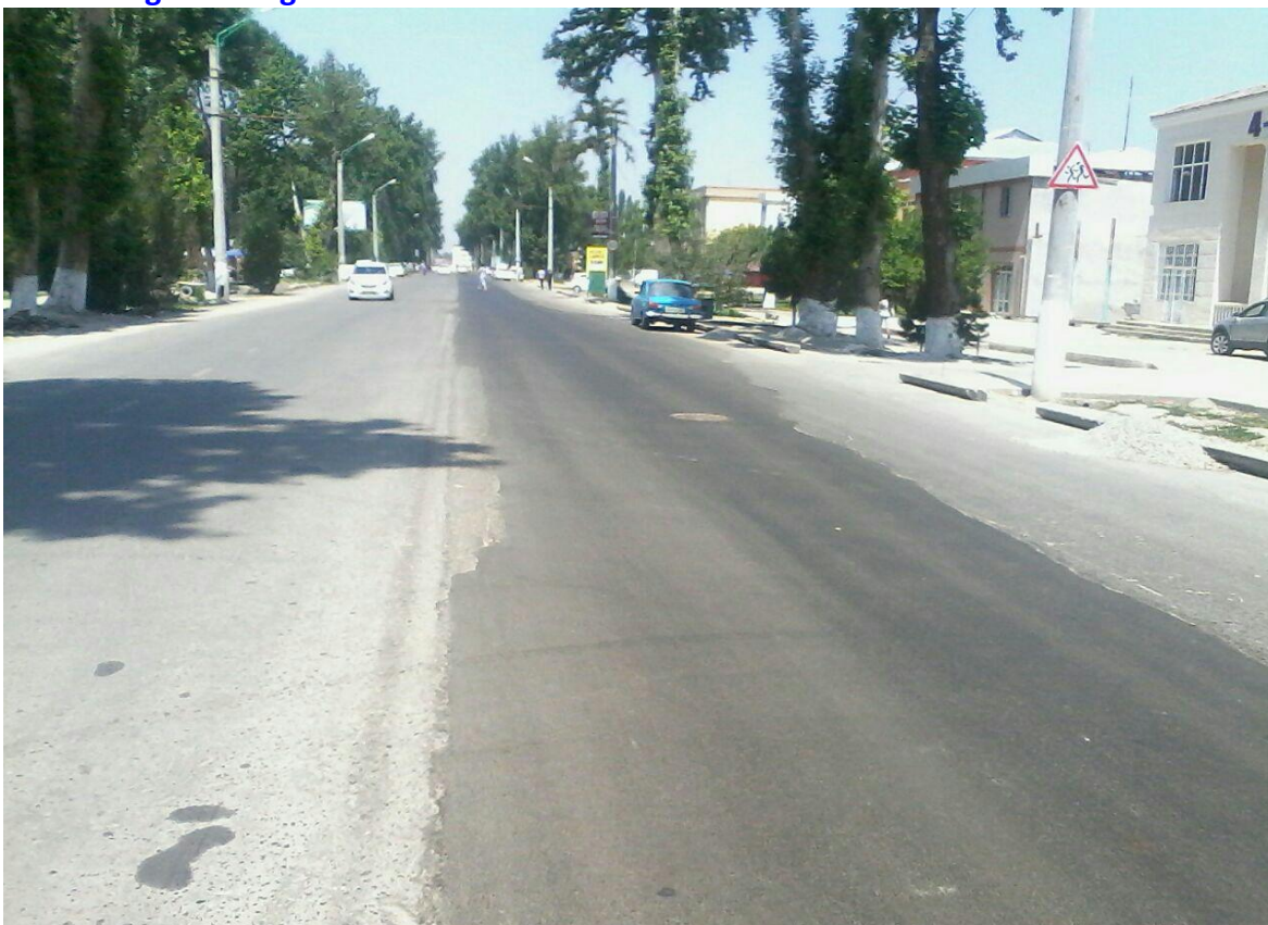
Corridors of the water supply pipes restored with asphalt cover satisfactorily
