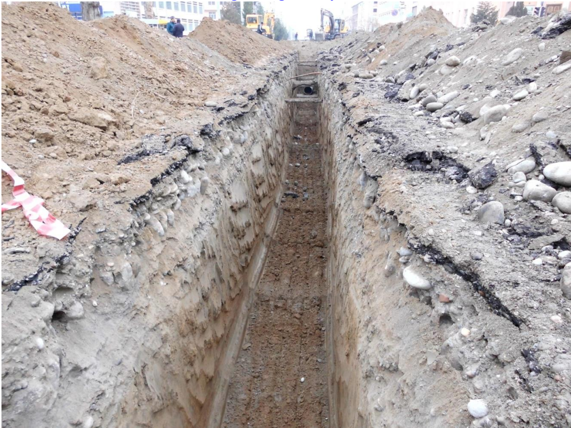
Excavate a trench for networks in Fergana city
