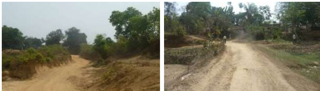
Existing Condition of the Road
