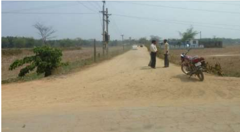
Starting Point of corridor
