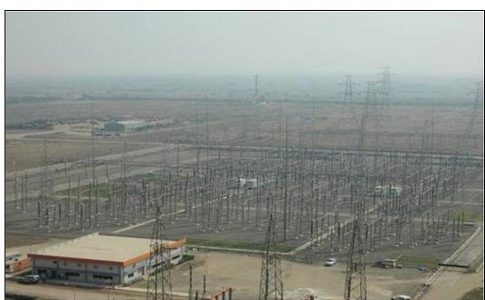
Figure 2-9: Typical 400kV switch yard
