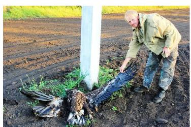
Figure 6-1 : Bird electrocution with transmission line
