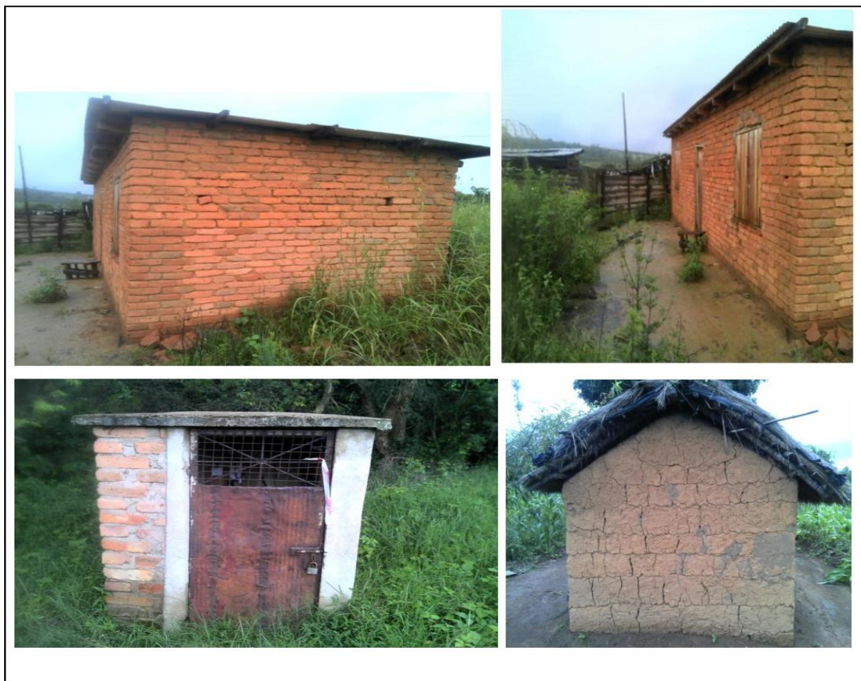
Figure 7: Some of the Houses located in the Transmission Corridor
