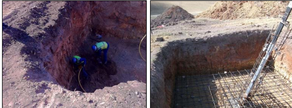
2 Figure 2-8: Preparation of tower foundation and tying of steel reinforcement
