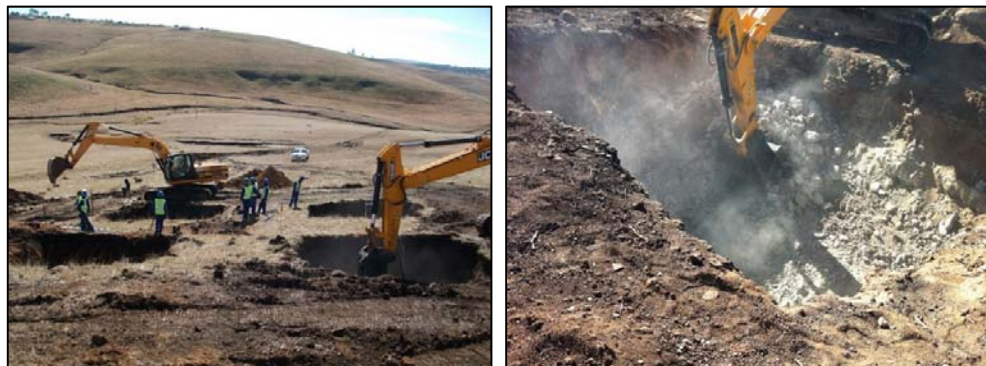
1 Figure 2-7: Construction process of tower foundations
