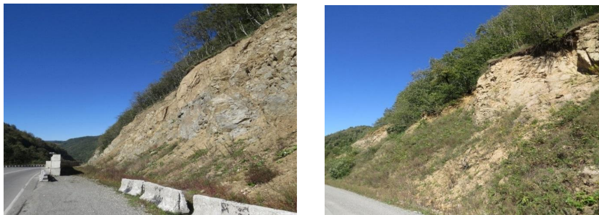
Figure 6.3.3. Slumping landslide segments on the left bank of the river
