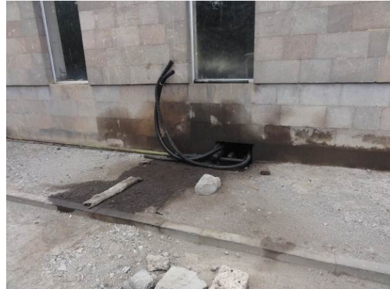
Photo 20: Oil leakages at oil refinery station
