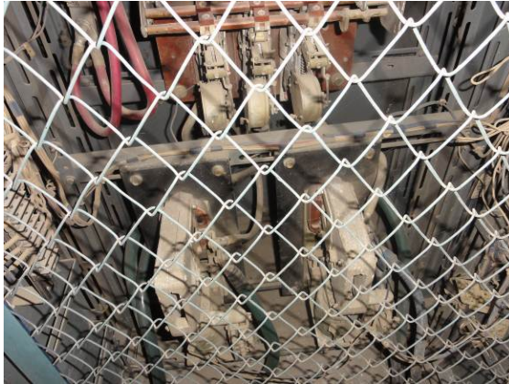
Photo 19: Asbestos plates inside electrical devices
