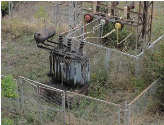
Photo 12: Old leaking transformer without drainage system
