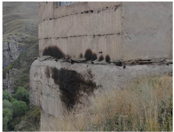
Photo 6: Oil leakages at outlet control building
