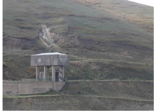
Photo 4: Erosion on slope above intake control building
