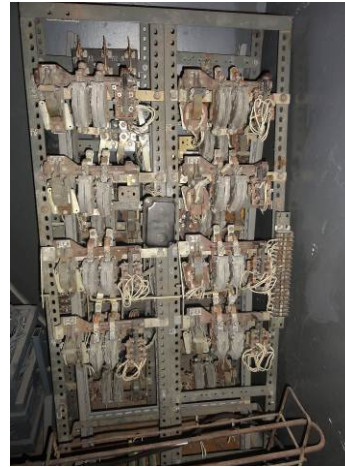
Photo 24: Asbestos plates inside electrical devices
