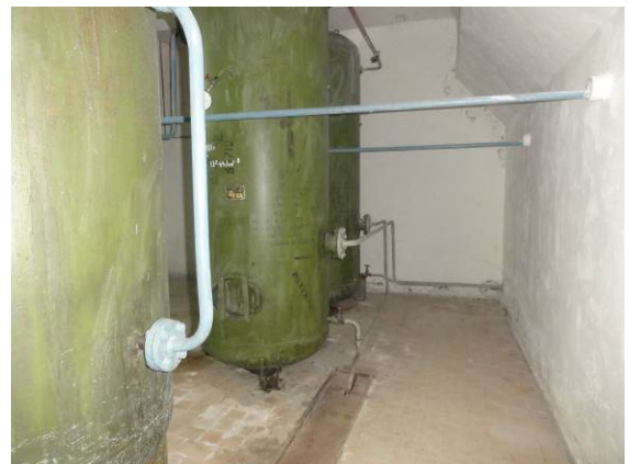
Photo 18: Oil-water mix from tanks is led to river
