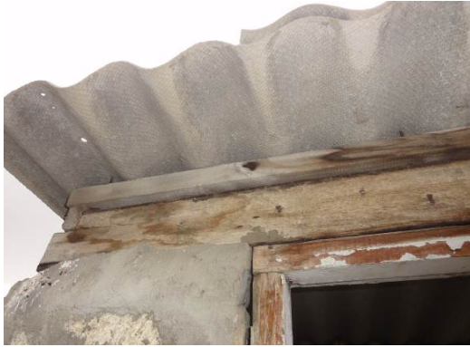
Photo 3: Eternit roof of pit latrine probably containing asbestos
