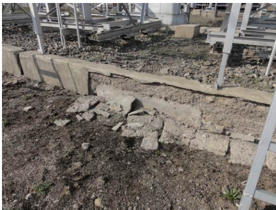
Photo 17: Broken spill wall below circuit breakers
