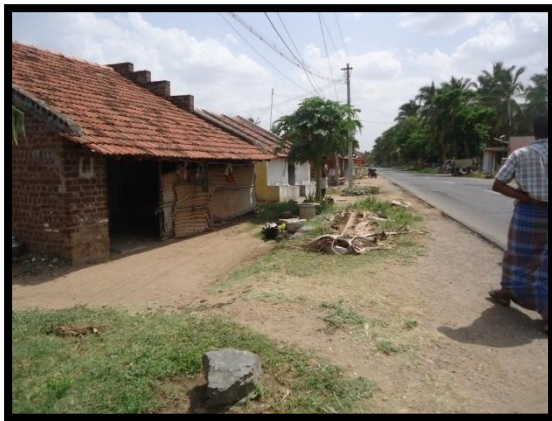
Residence cum Commercial - Major - Encroacher Km 51.605 - SH79 - LHS Col - 11.7 - Offset 8.0m - RoW 11.0
