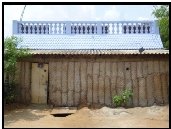
Residence - Major - Encroacher Km 48.55 – SH37 - RHS Col – 14.43 - Offset 6.7M - RoW 10.72
